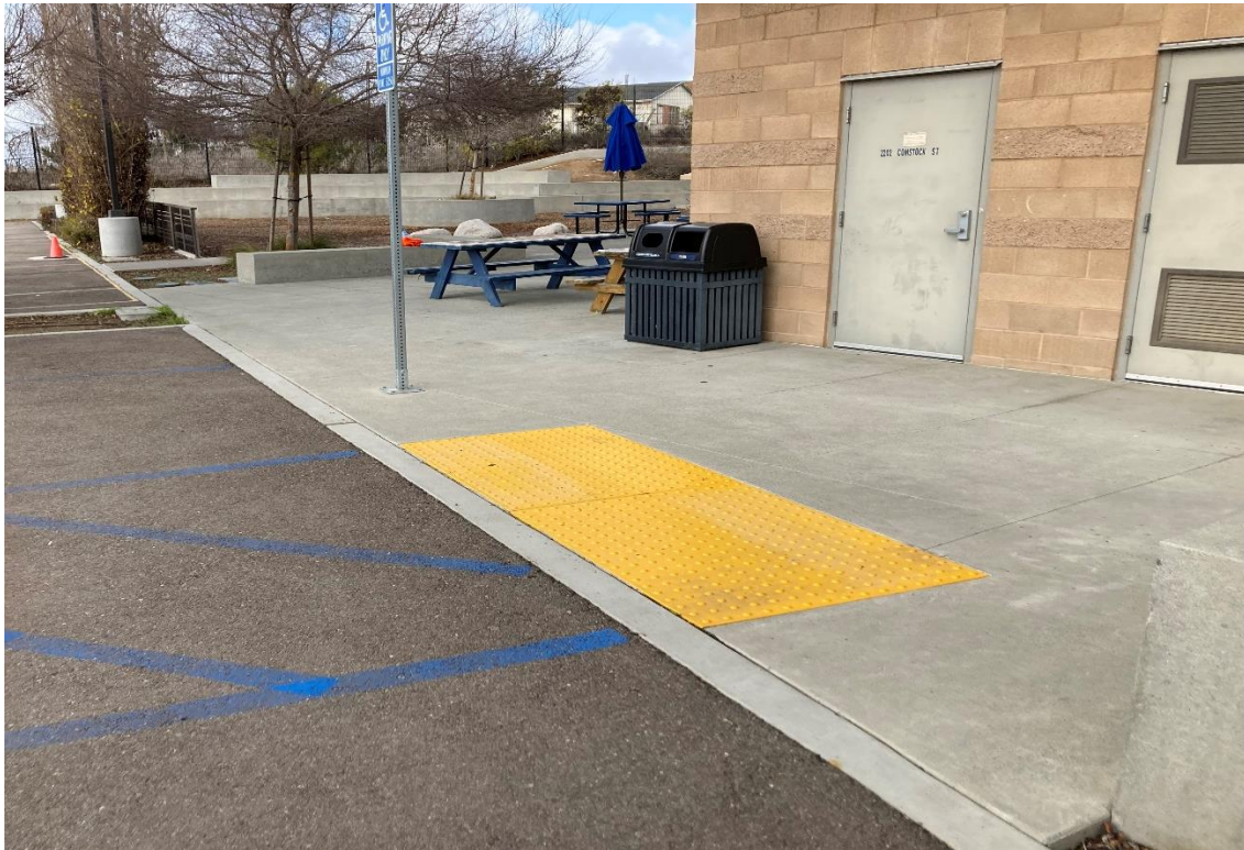
PHOTO 2 – Location where (2) ADA compliant gates are to be installed.
