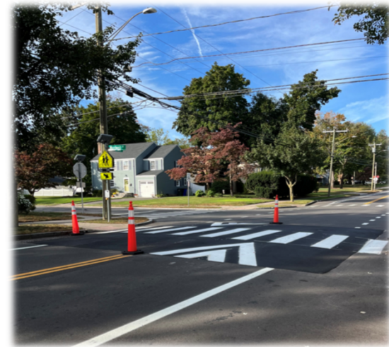
Boulevard at Wardwell Road Raised Crosswalk
