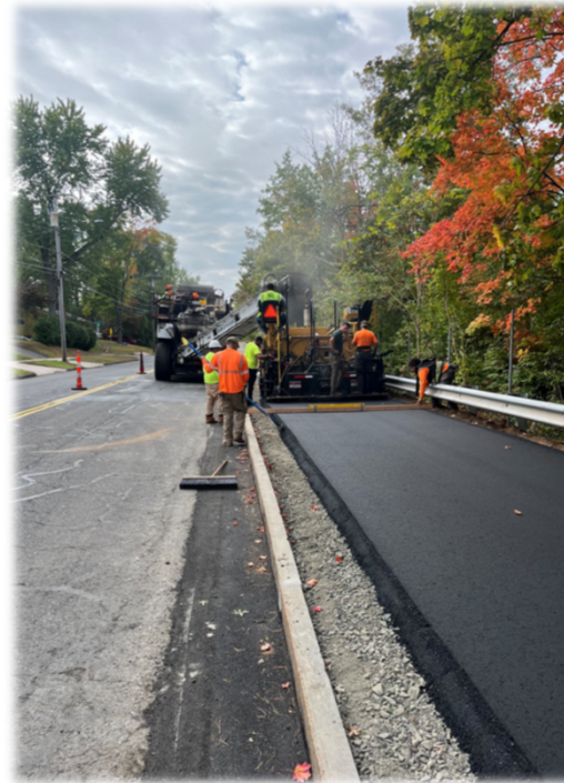
Trout Brook Trail - Phase 3 Under Construction
