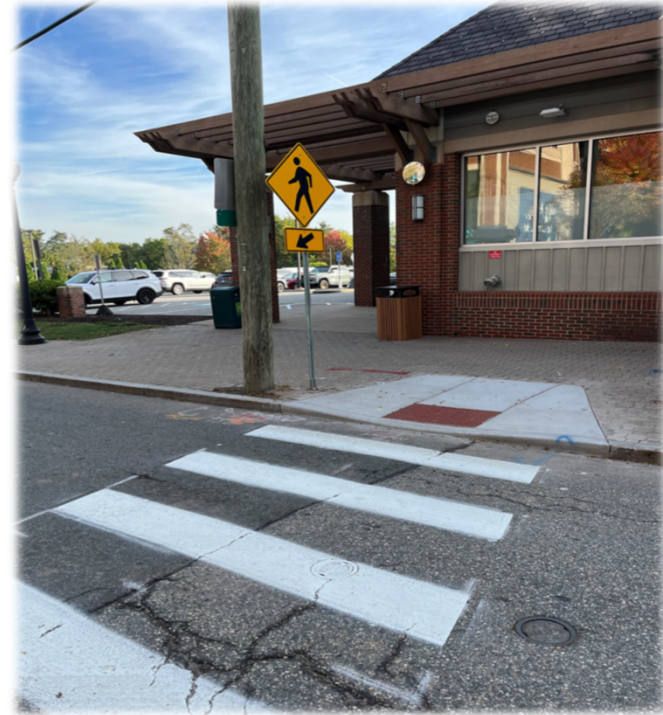
Raymond Road New Sidewalk Ramp
