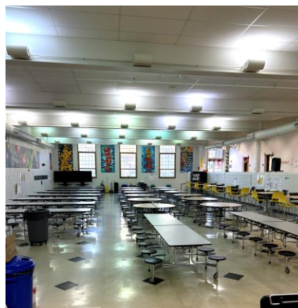
Water infiltration reported in cafeteria
