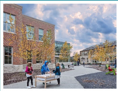
Barrington Elementary School Renovation & Addition
