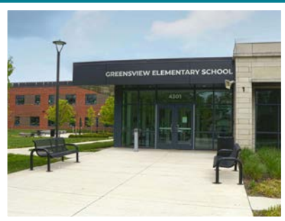
Greensview Elementary School Rebuild
