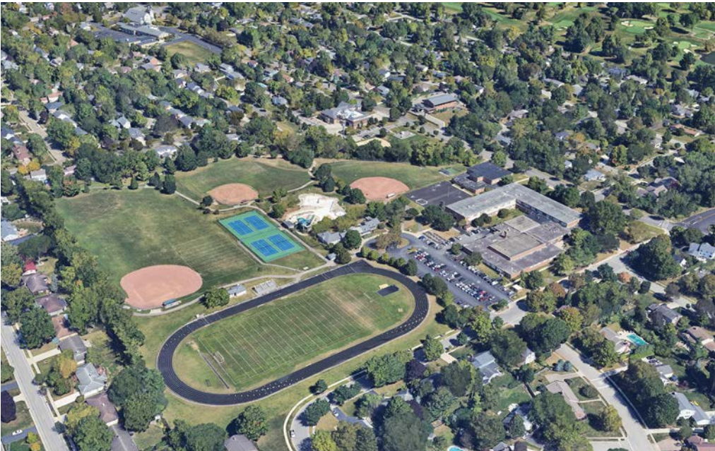
Hastings Middle School View from Southwest
