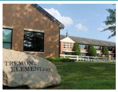
Tremont Elementary School Renovation & Addition
