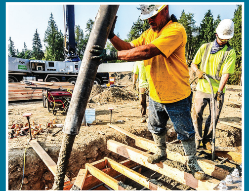
Concrete pour at New Elementary School in Redmond Ridge
