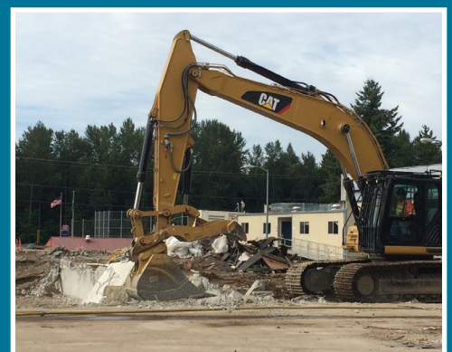
Juanita High School demolition
