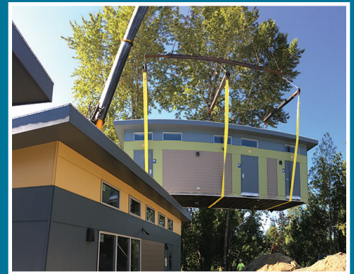
Modular unit being lowered into place at Explorer Community School
