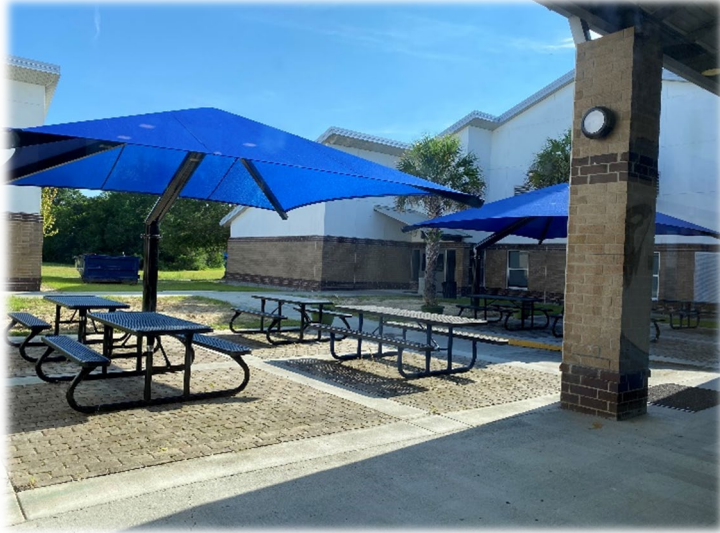
Outdoor dining shade structures at Whale Branch Middle
