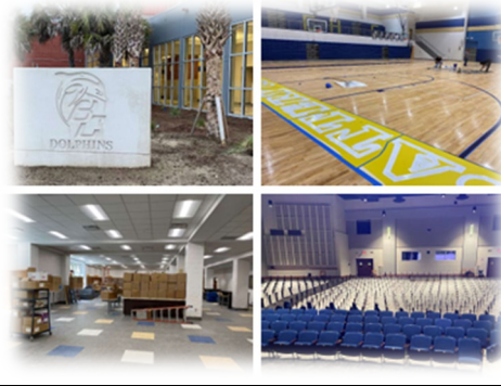
Renovation of Battery Creek High School
