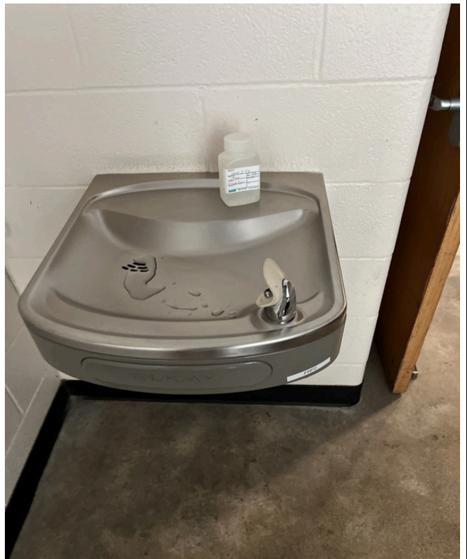
7/8/2024 - 13001-2 - Fleetridge Elementary - South Entrance Outside Gym
