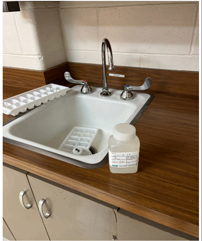
7/8/2024 - 13001-10 - Fleetridge Elementary - Clinic Sink
