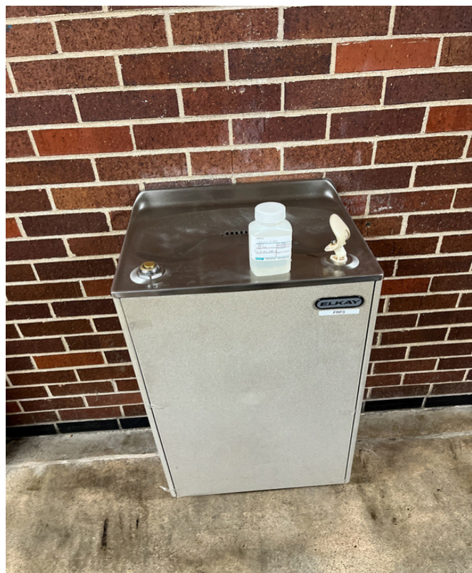
7/8/2024 - 13001-3 - Fleetridge Elementary - Outside Main Restroom
