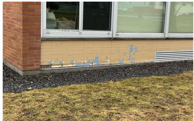
Failing Masonry
