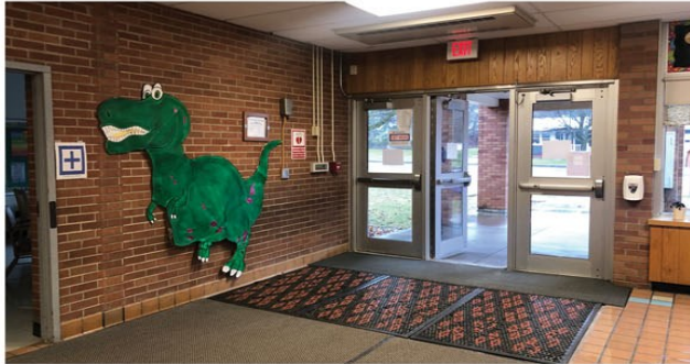
Create New Secure Entry Vestibule
