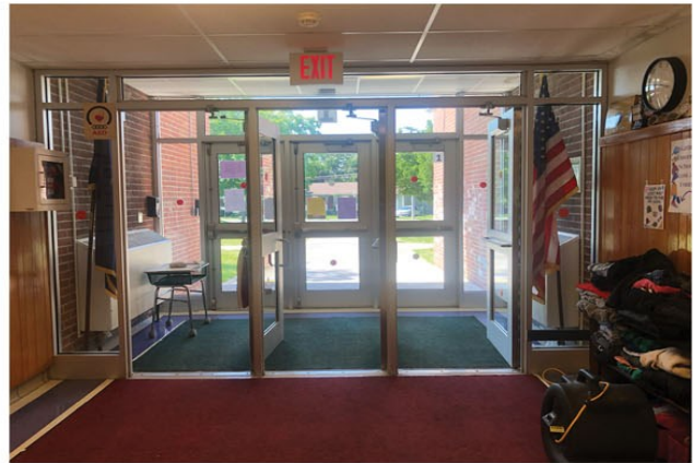
Create New Secure Entry Vestibule
