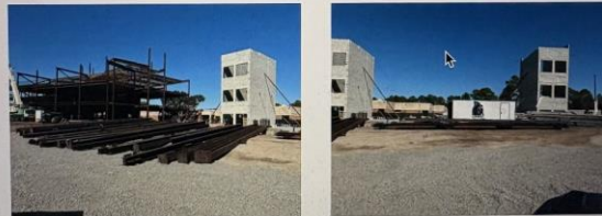
Steel erection in progress. Masonry Stair towers
