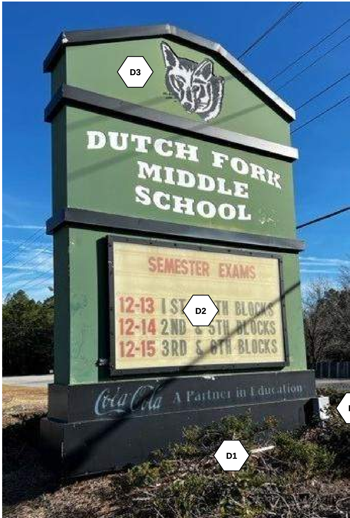
6 VIEW OF SIGN EXISTING CONDITIONS A-201
