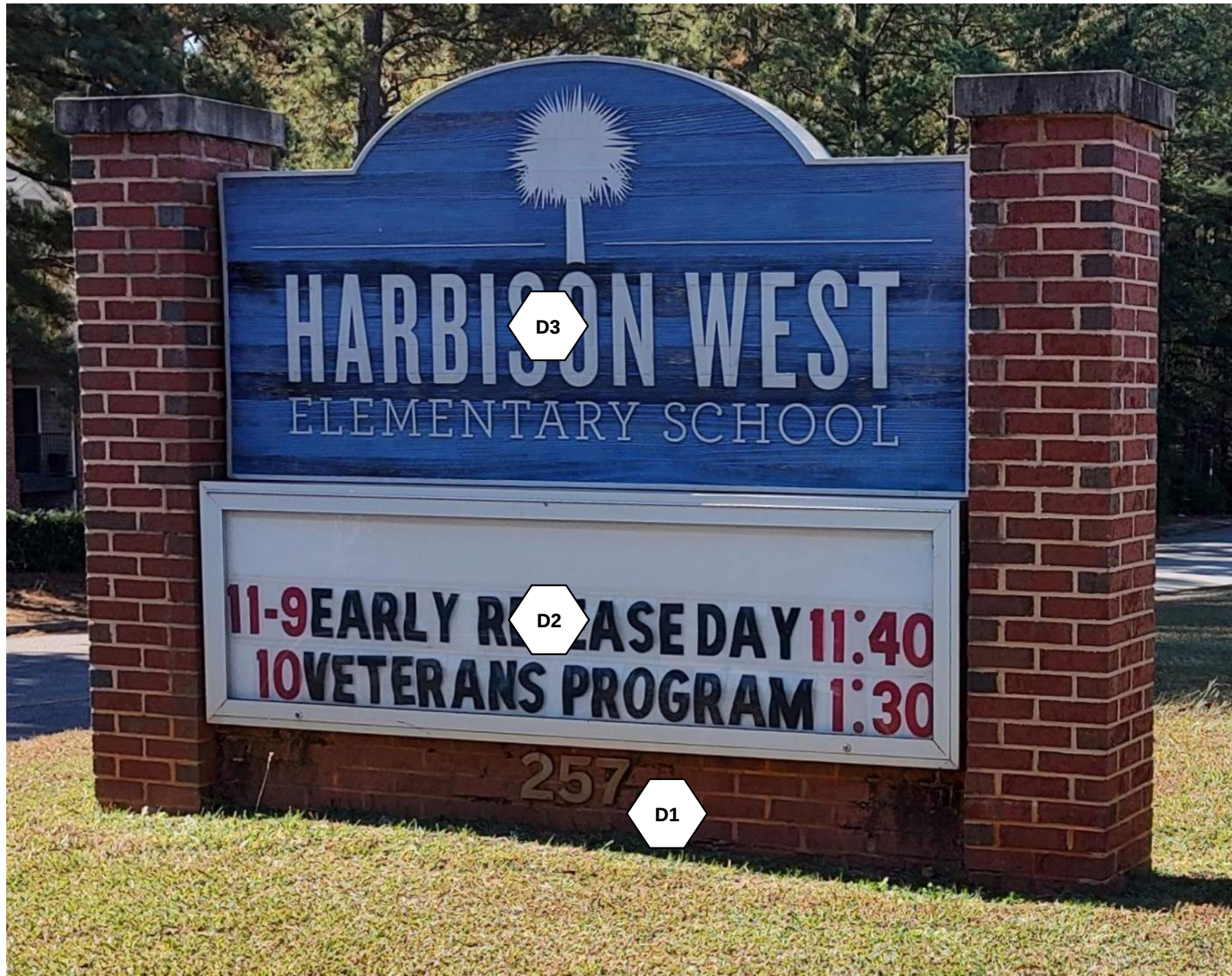
6 VIEW OF SIGN EXISTING CONDITIONS A-203
