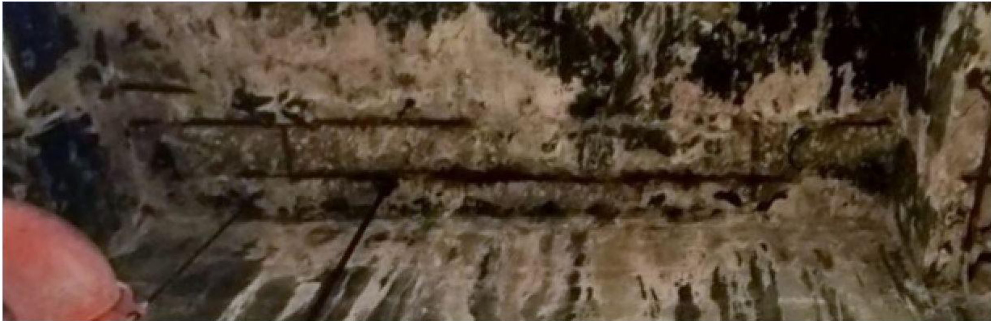
1 TYPICAL SLAB UNDERSIDE SPALL REQUIRING REPAIR NO SCALE
