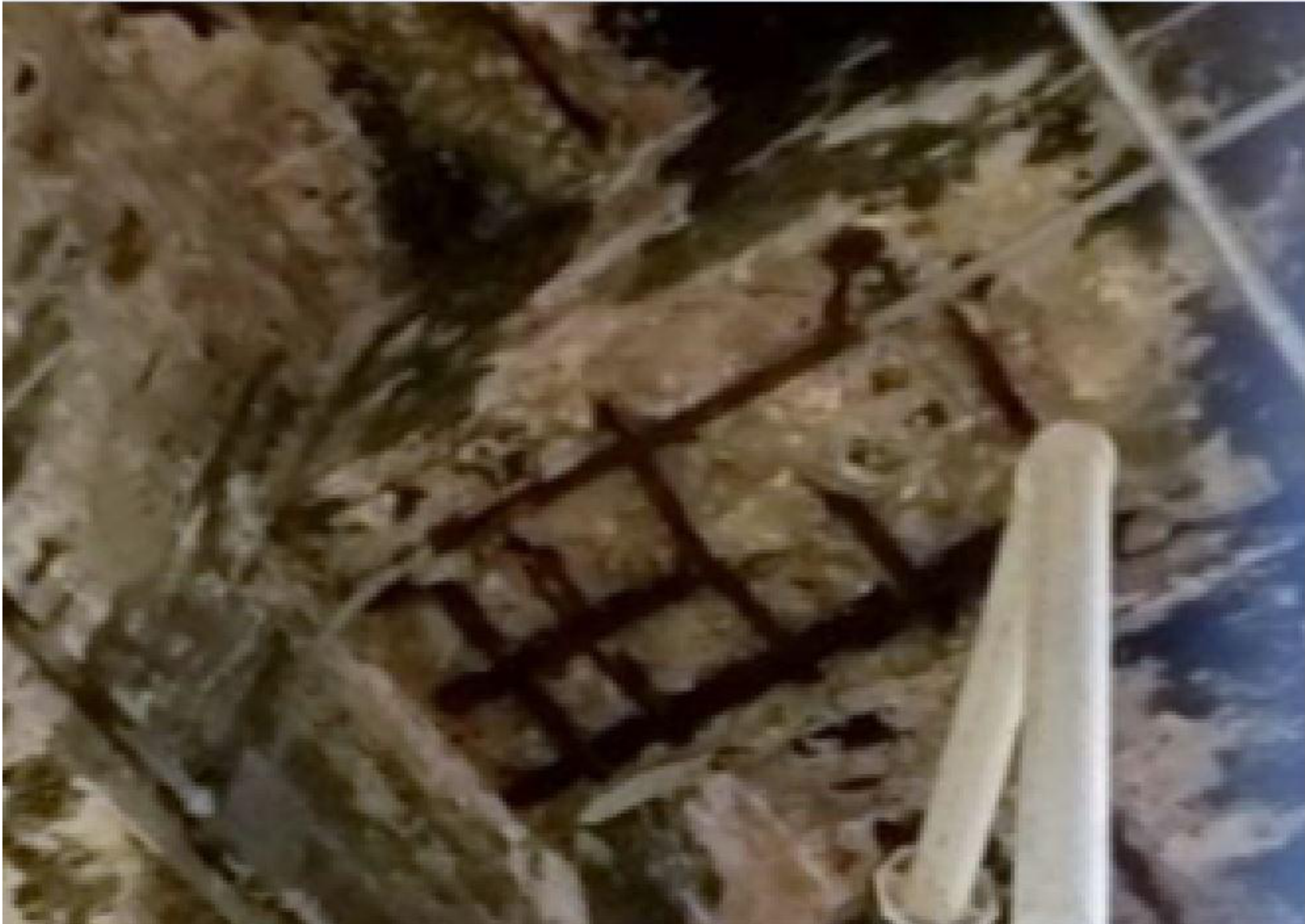
2 TYPICAL BEAM UNDERSIDE SPALL REQUIRING REPAIR NO SCALE
