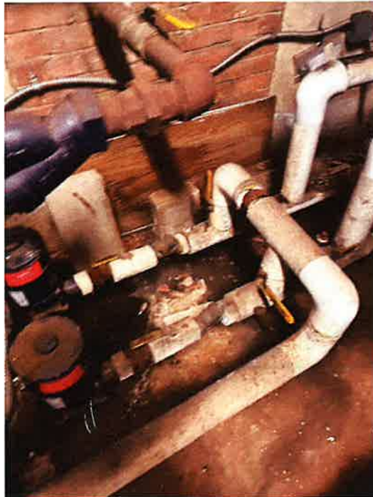
Photo 1: Condensate Insulation
