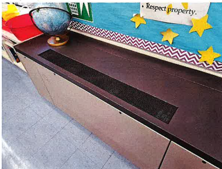
Photo 10: Unit Ventilator
