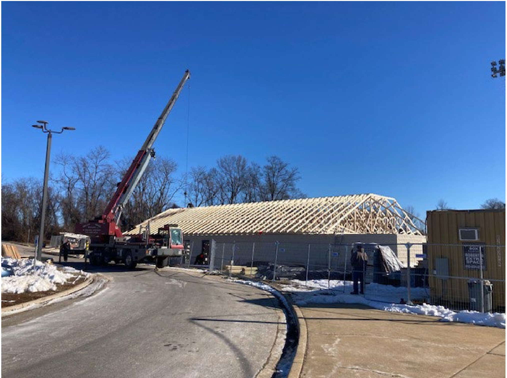
PERRYVILLE HIGH SCHOOL – FIELDHOUSE
