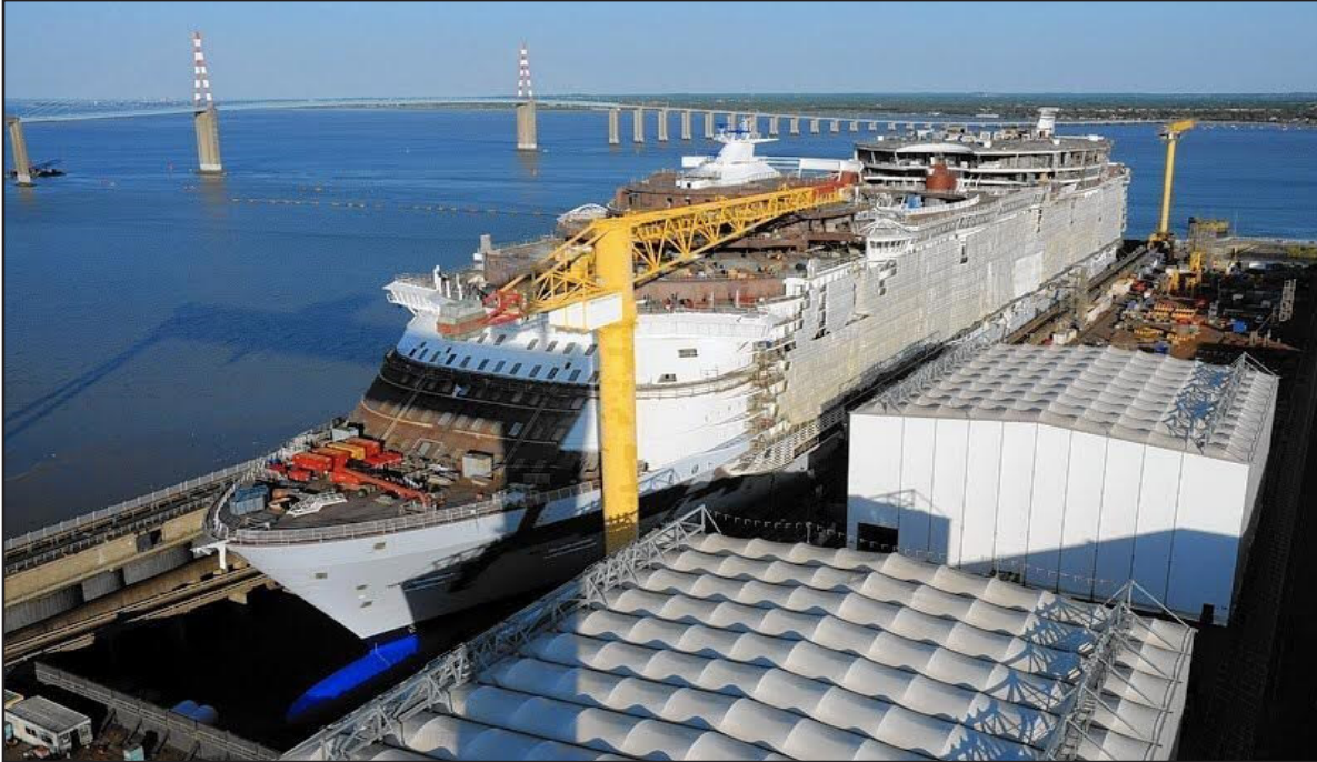
The Harmony of the Seas construction in process.
