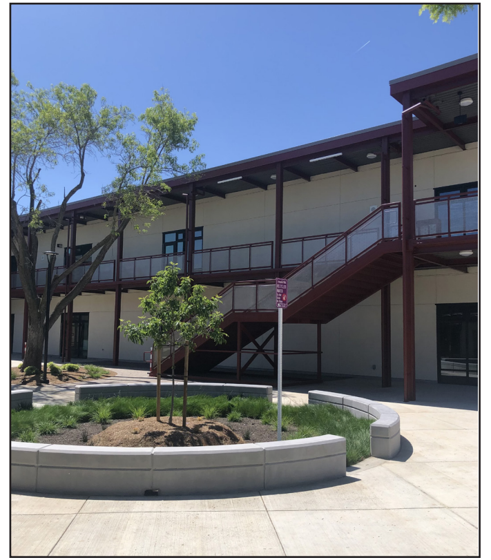
The new B and C buildings on campus are finally open for students and staff to work inside. New landscaping, an elevator, and staff work space are just a few of the features. Photo by Ayden Curameng
