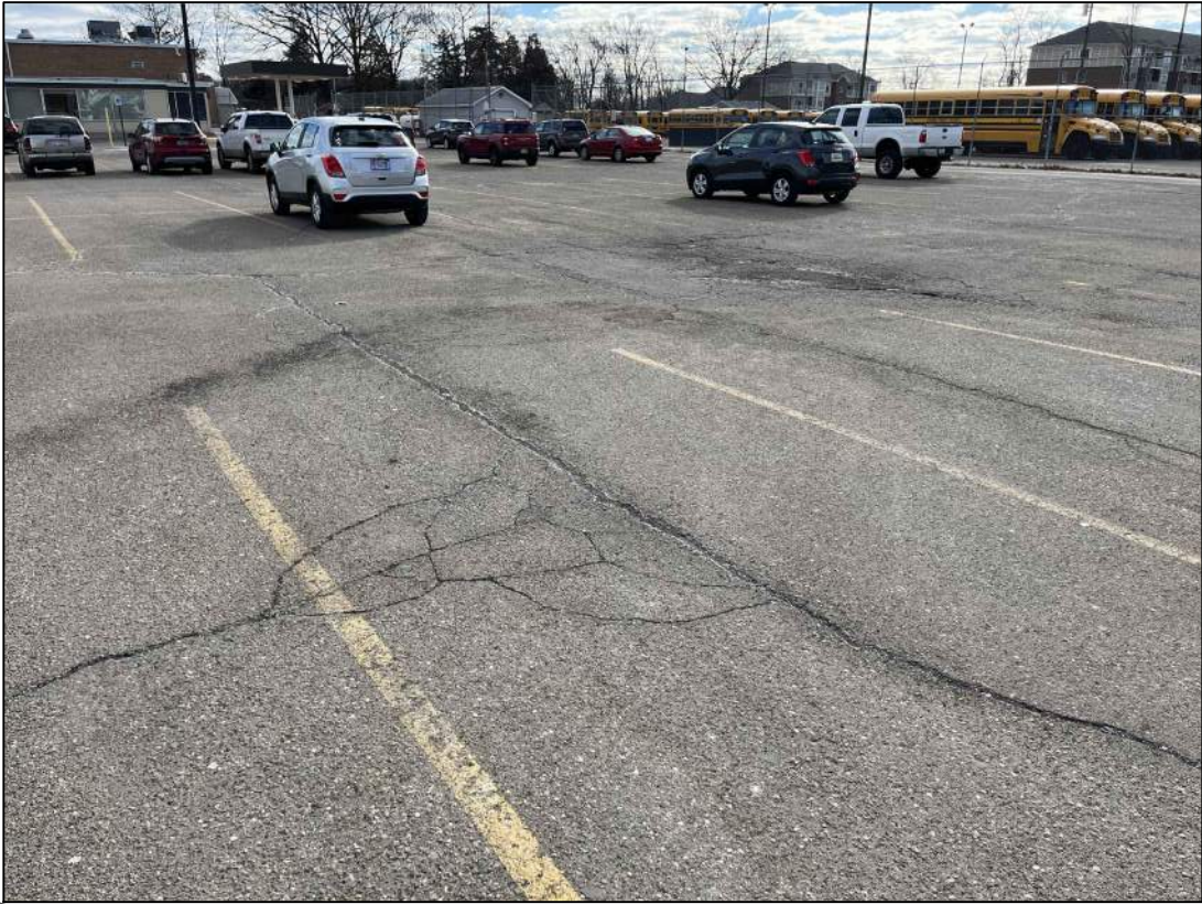
3 Block Cracking - Alligator Cracking - Potholes NTS
