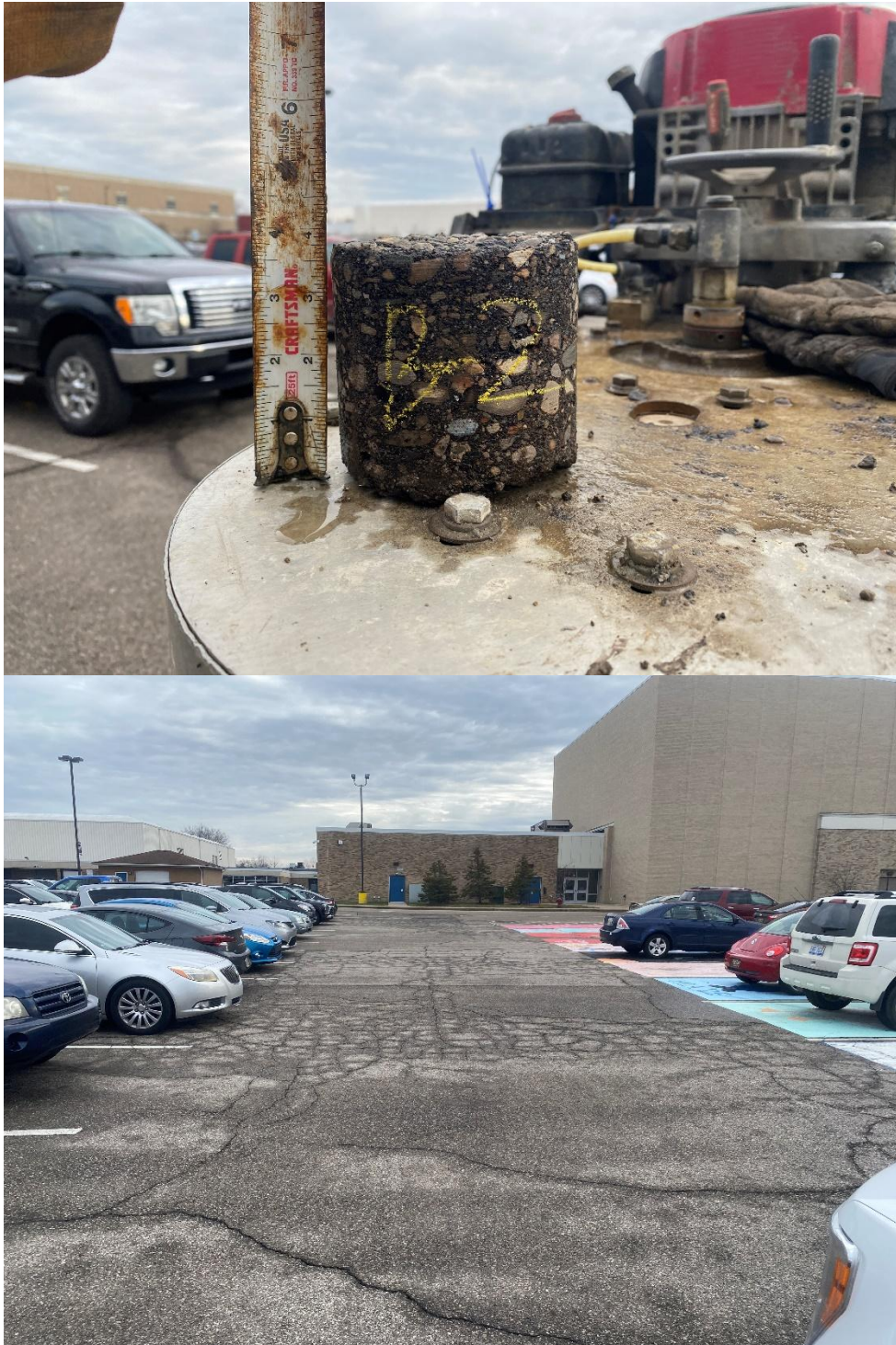
Photo Nos. 3 and 4 – Pavement core and surface conditions at B-02. Pavement distress consisting of high-severity fatigue and transverse cracking, and low-severity longitudinal cracking. View to the east.
