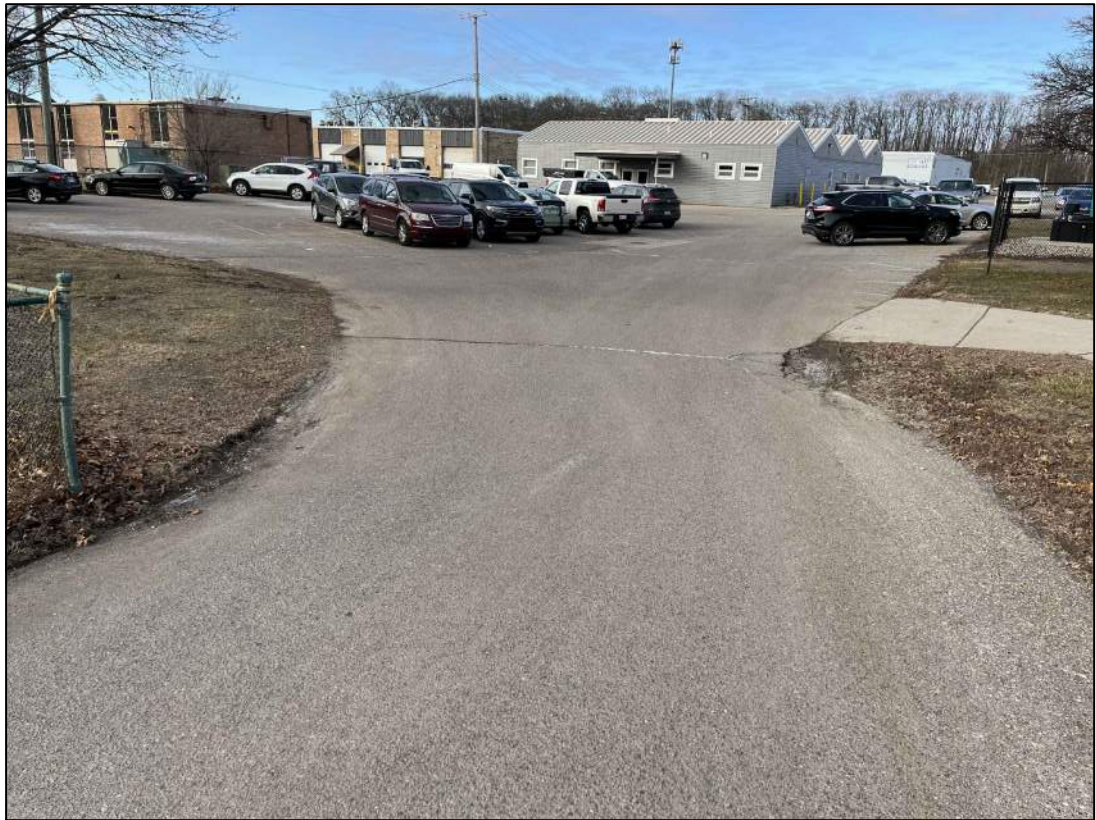
2 Transverse or Joint Cracking NTS
