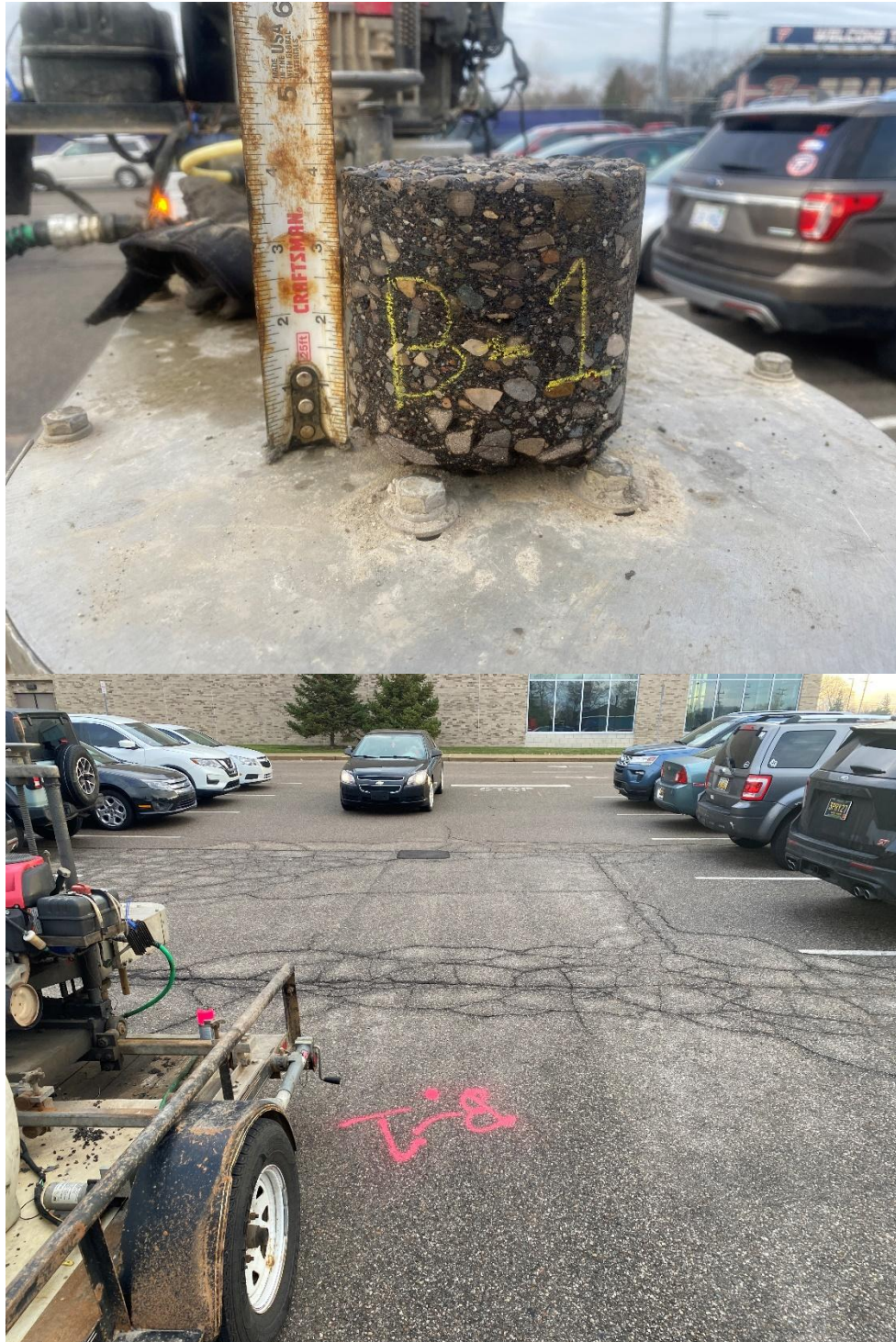
Photo Nos. 1 and 2 – Pavement core and surface conditions at B-01. Pavement distress consisting of medium-severity fatigue cracking, and low-severity transverse and joint cracking. View to the east.
