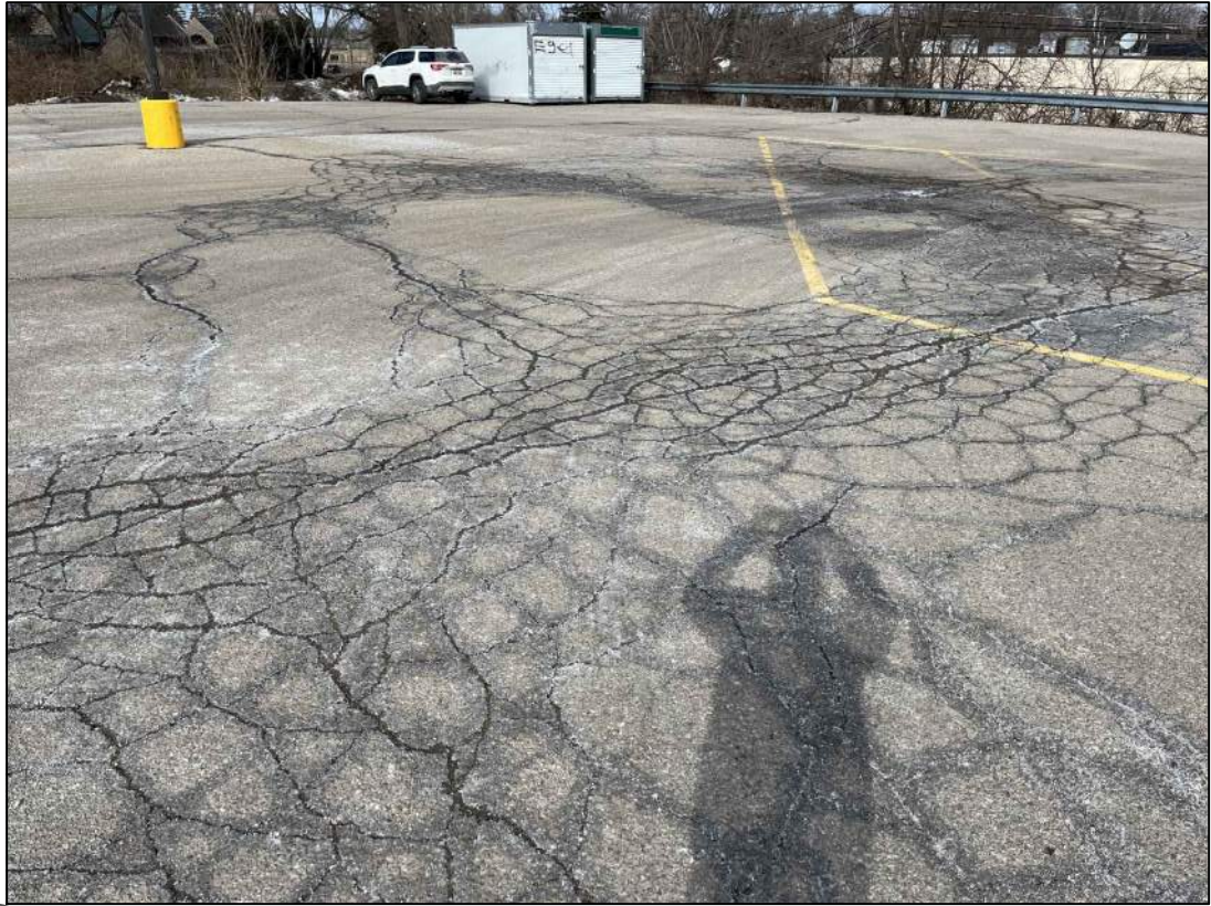
2 Block Cracking - Alligator Cracking NTS
