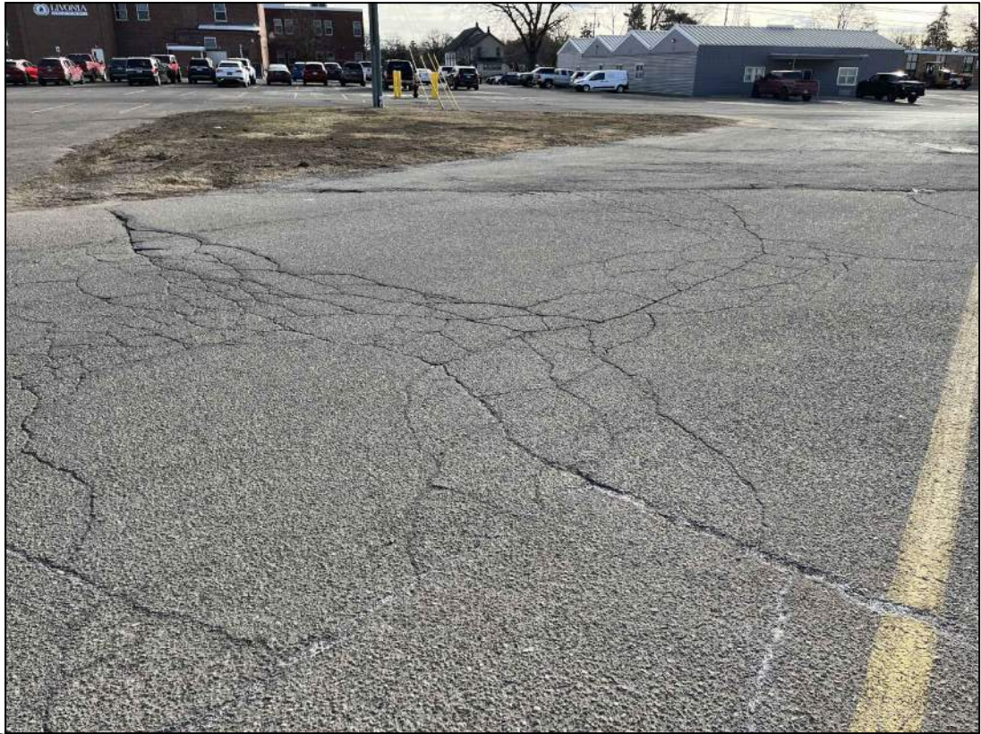
1 Block Cracking - Alligator Cracking NTS
