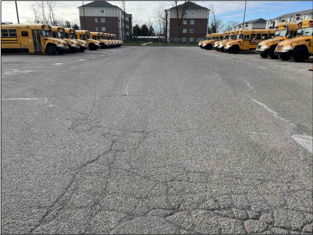
3 Alligator Cracking NTS
