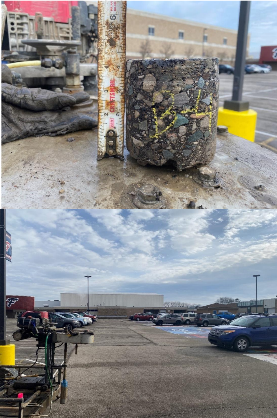
Photo Nos. 7 and 8 – Pavement core and surface conditions at B-04. Pavement distress consisting of medium-severity fatigue cracking and low-severity transverse cracking. View to the east.
