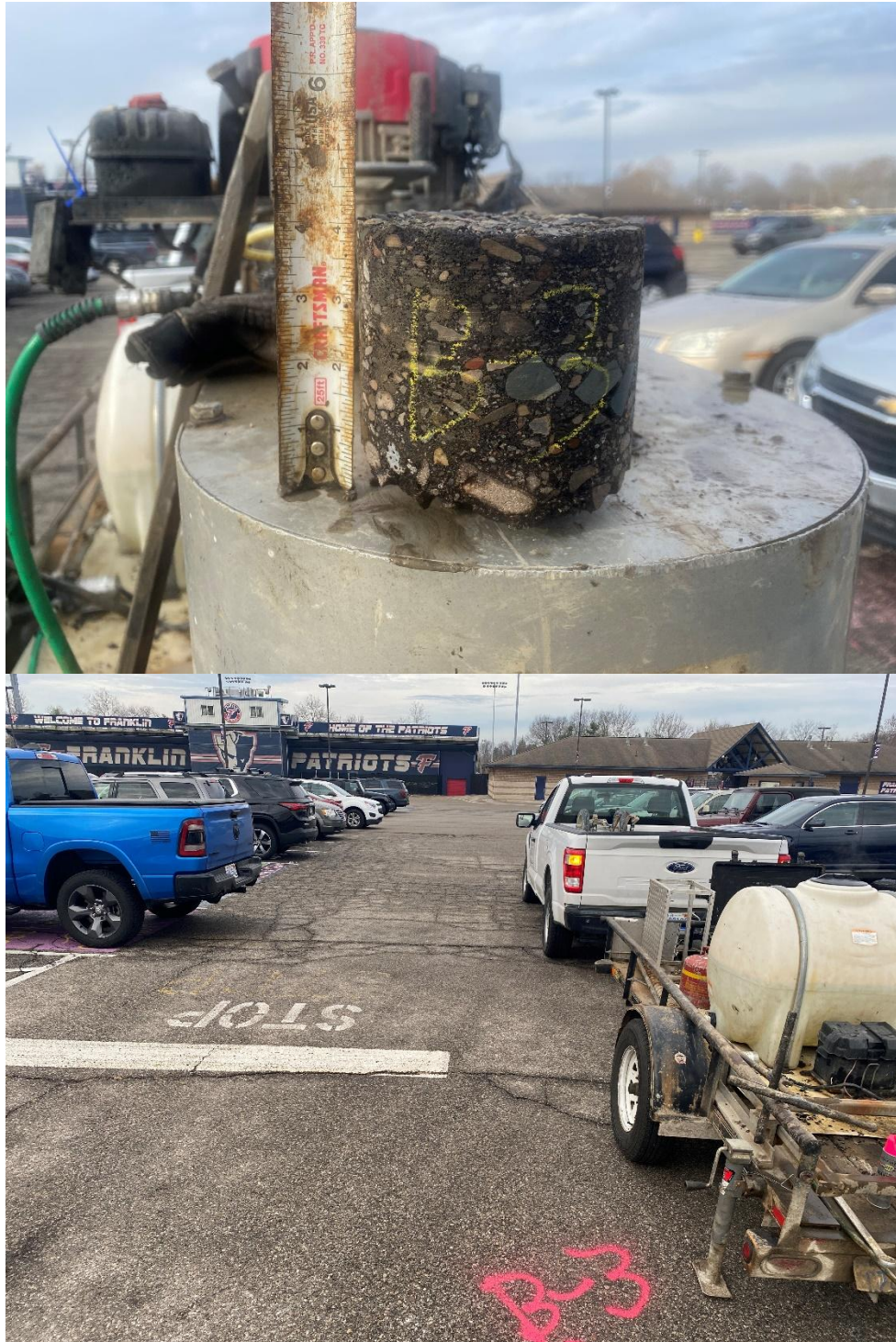
Photo Nos. 5 and 6 – Pavement core and surface conditions at B-03. Pavement distress consisting of high-severity fatigue cracking and medium-severity transverse cracking. View to the west.
