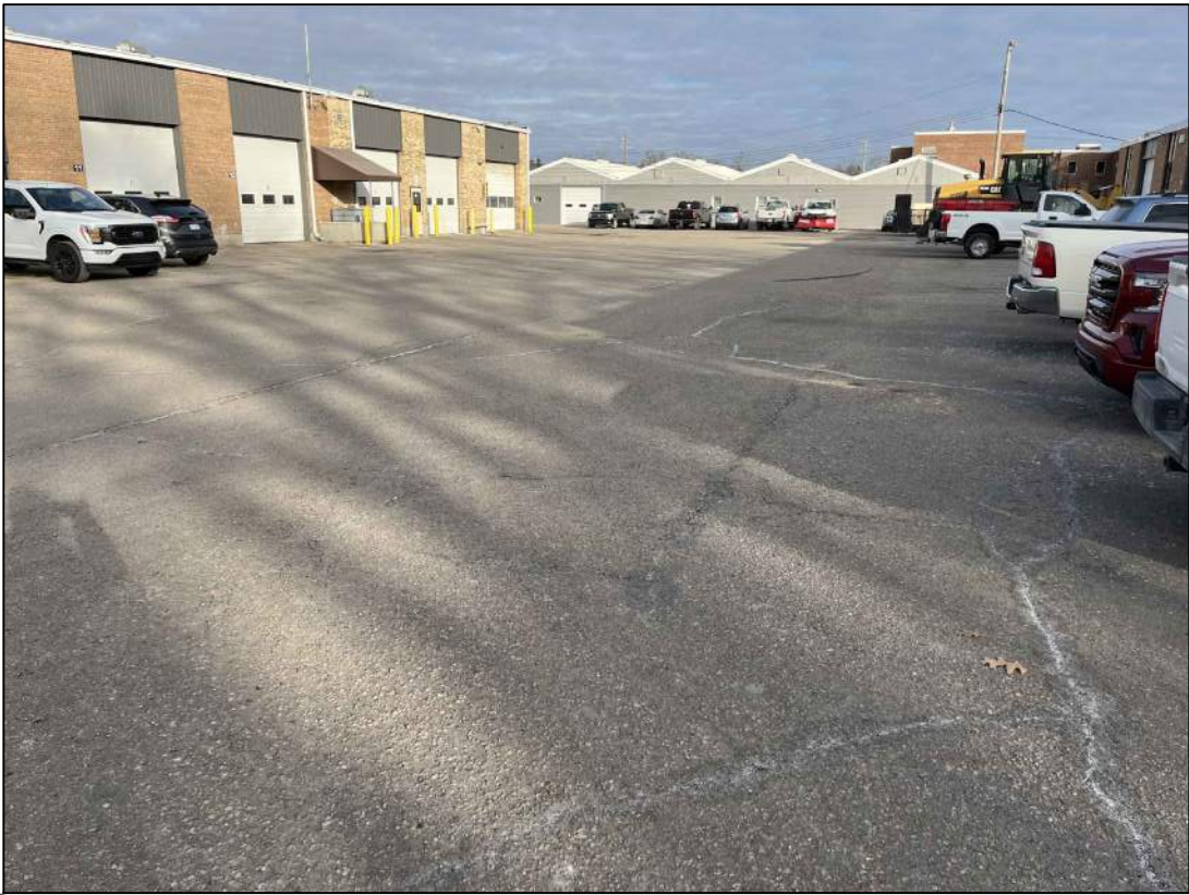
3 Negligible to Low-Severity Block Cracking NTS
