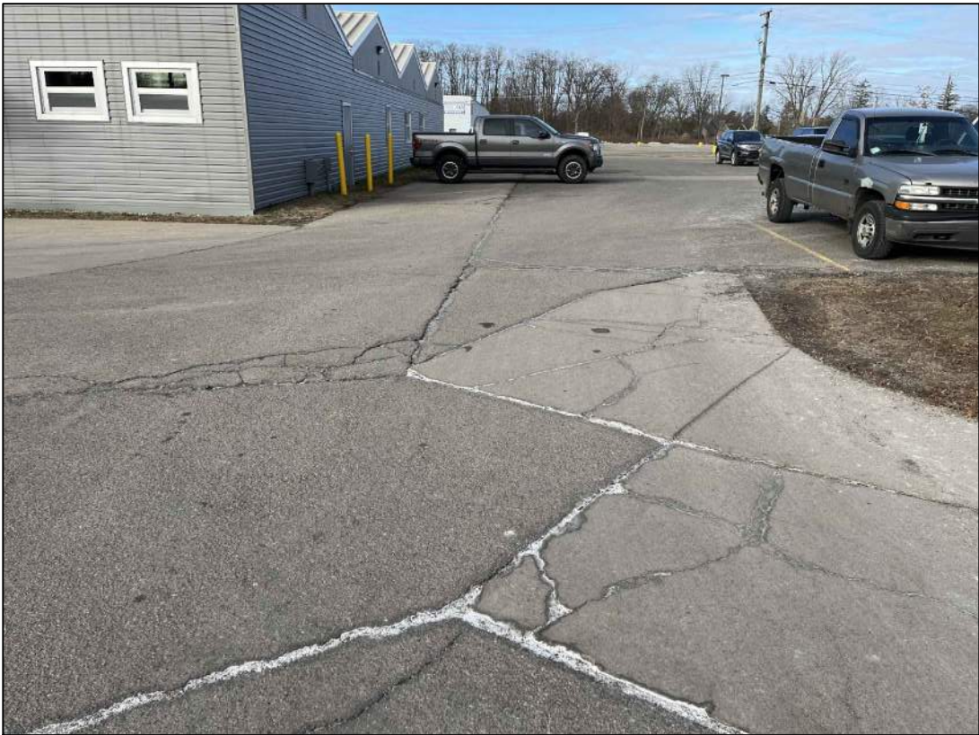
3 Alligator Cracking - Salt Buildup NTS
