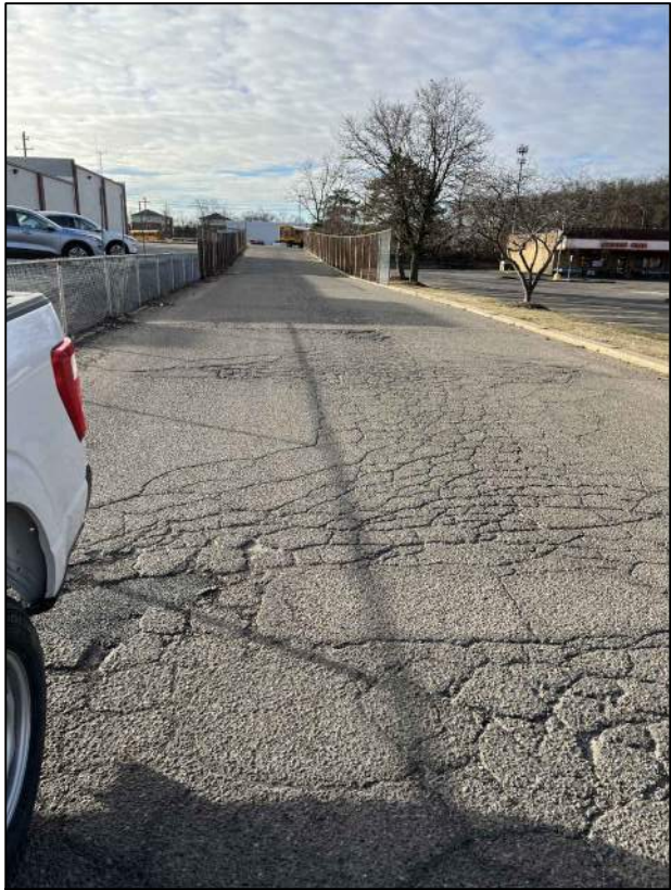
1 Alligator Cracking
