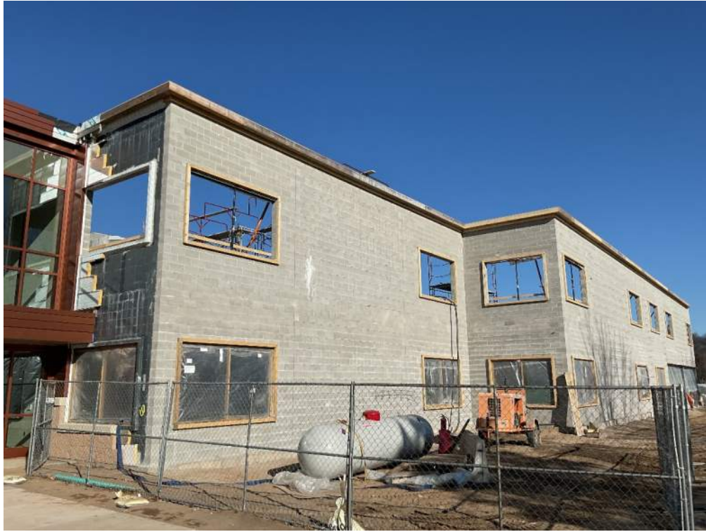
Classroom Addition 2 nd Level CMU, Window Blocking, and Roof Edge
