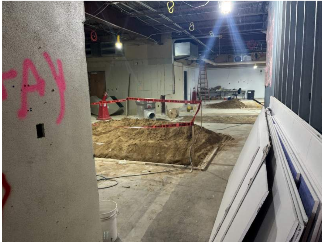
Segments E&F – Former Admin Area Underground MEP Work
