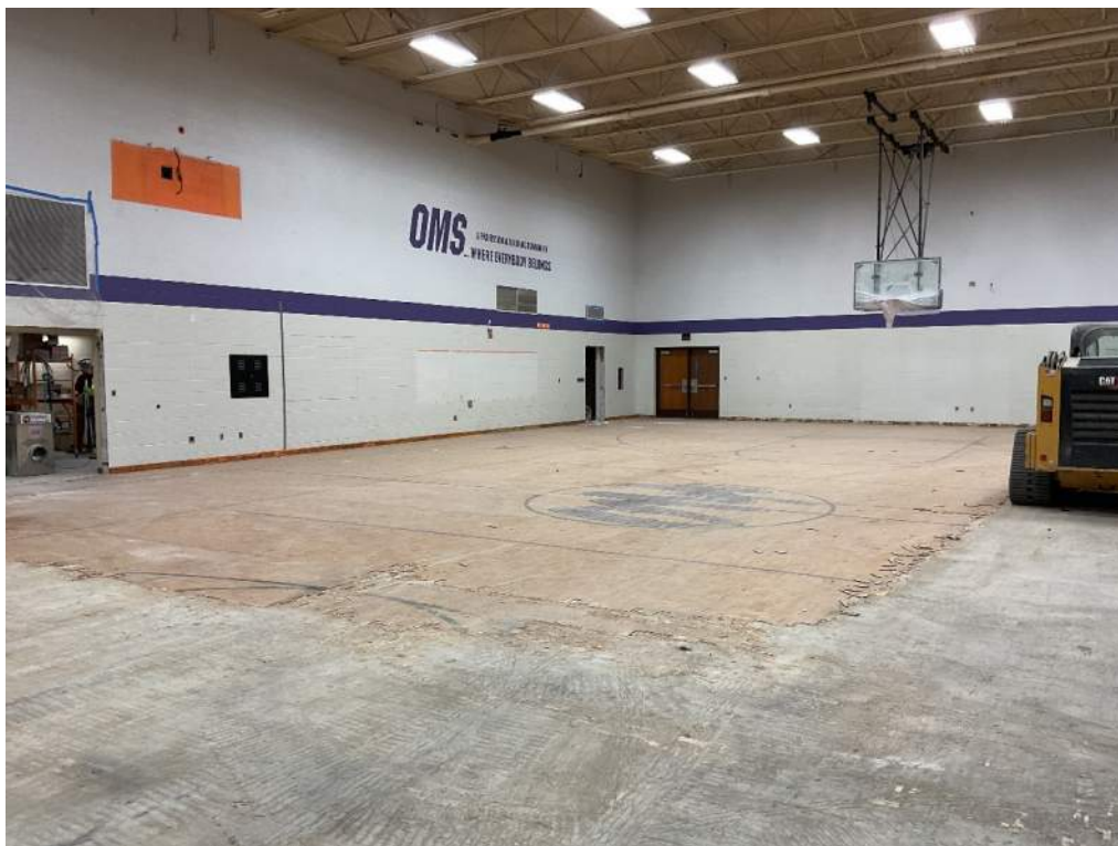
GYM 177 Old Gym Floor Demolition
