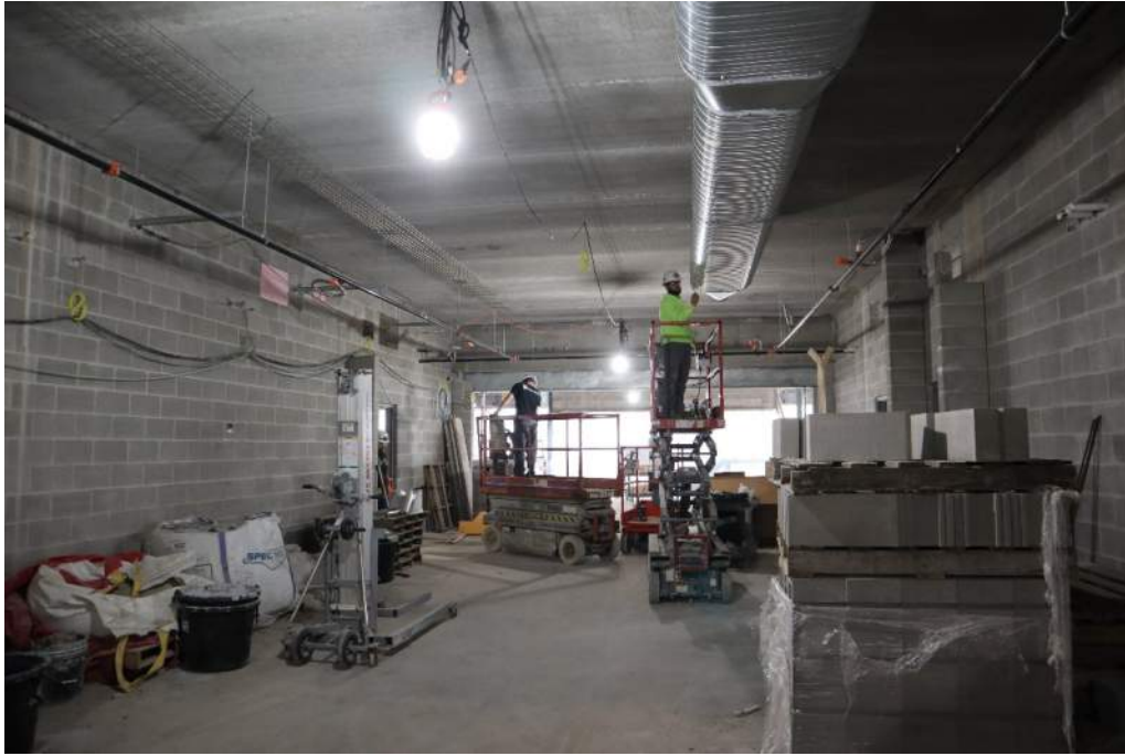
Segment F (Classroom Addition) Overhead MEPFS Rough-ins
