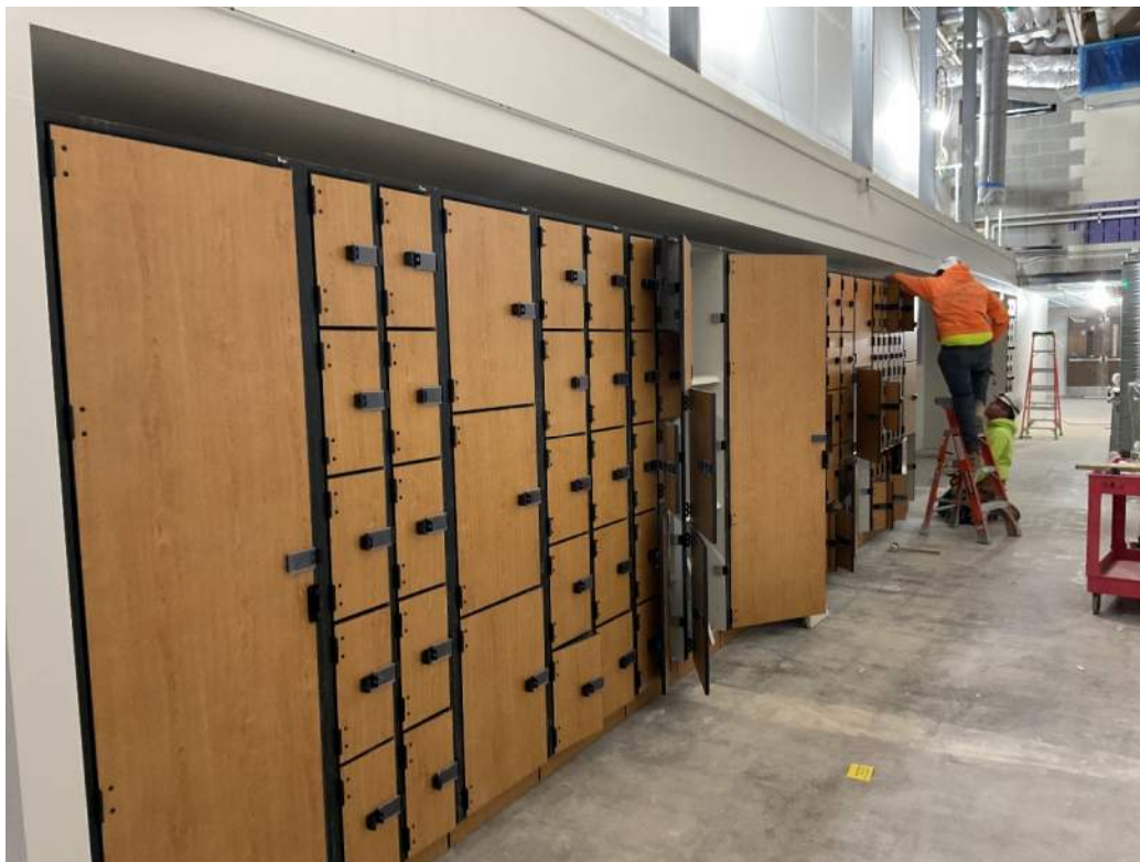
Segment A – New Instrument Casework Install
