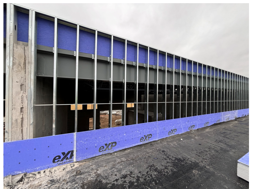
COLD FORM METAL FRAMING INSTALLED
