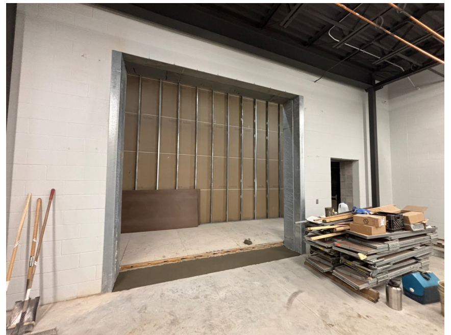
LAST OVERHEAD DOOR OPENING PUNCHED IN GYM ADD.
