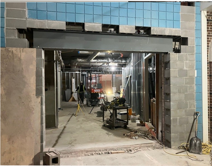
From top left, at Hidden River: Learning area terrazzo and glass installed; main-entry hallway lintel installed; mechanical and frame completed for inclusive toilet bank (January 2025)
