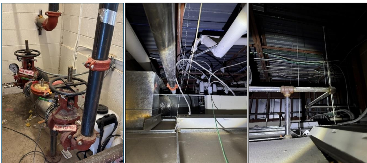
Figure 5.4. JMS Fire Sprinkler System Riser Room and Piping
