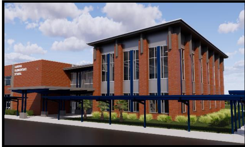
*Rendering represents design intent only and does not reflect final exterior finish selections*
