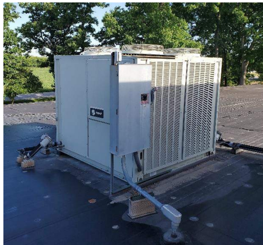
Photo 4: Condensing unit
