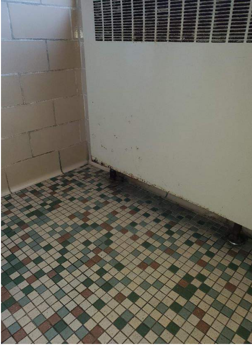
Photo 5: Floor beneath cabinet unit heater
