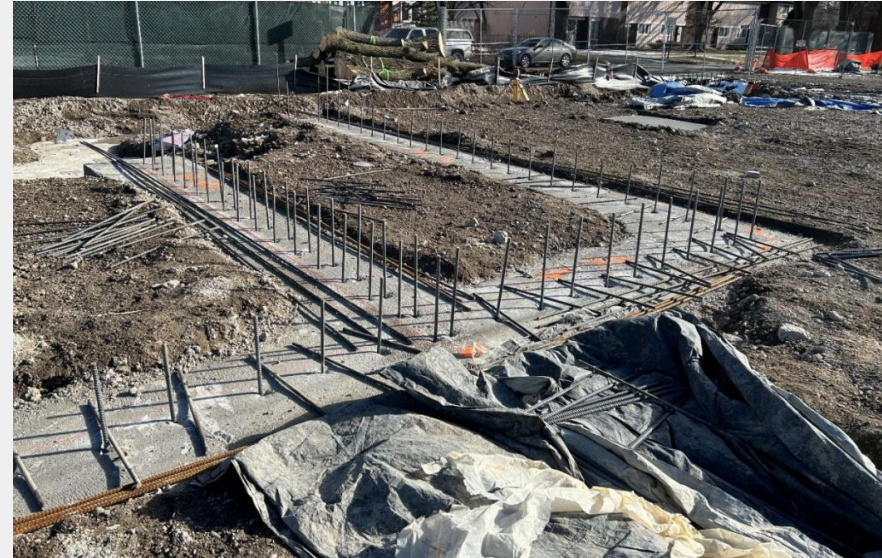
Foundation with rebar for the cafetorium (B. Kogan, 1/25)
