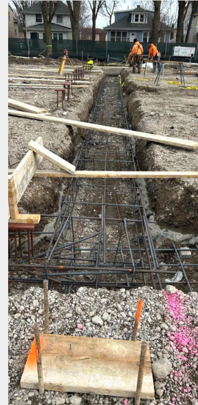
Foundation trench with rebar placed (B. Kogan, 12/24)
