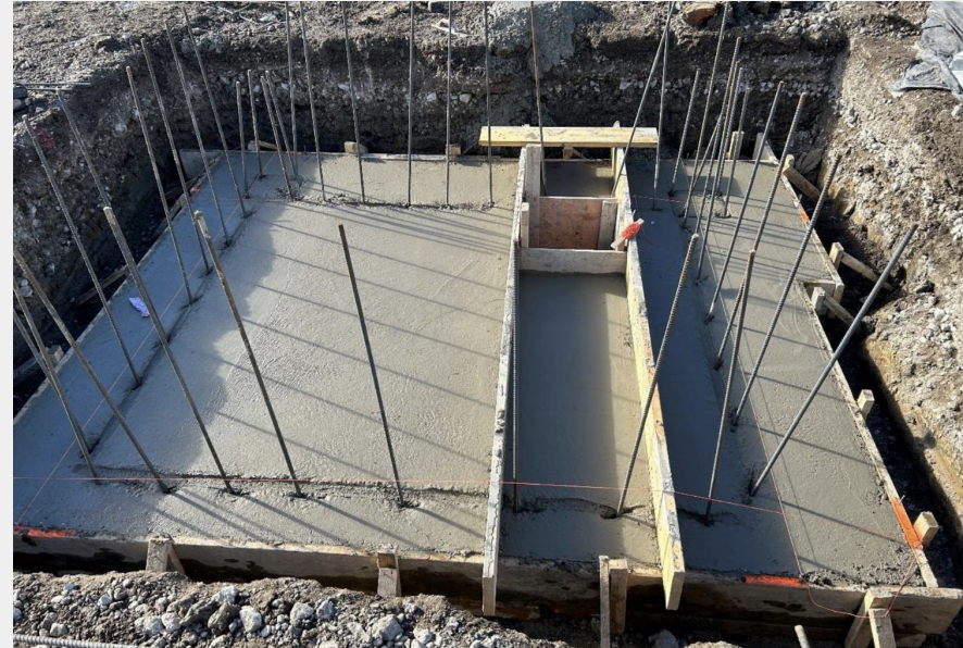
Foundation for the elevator shaft (B. Kogan, 1/25)
