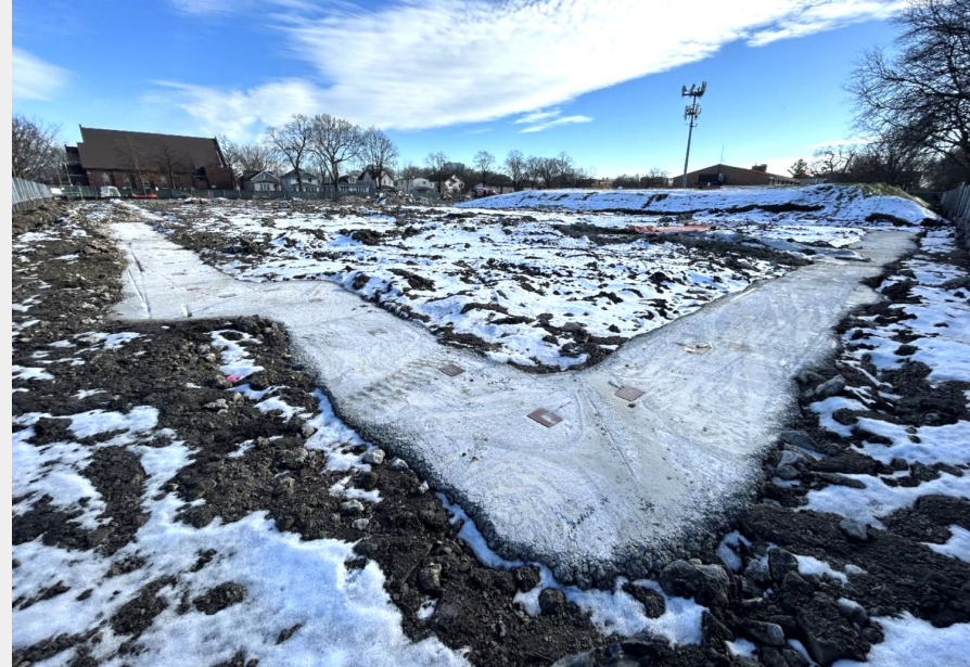
Foundation for northwest corner (B. Kogan, 1/25)
