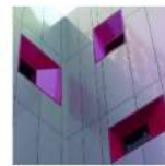
Kindergarten, Renovation - Paris, France. Evo Samuel Architect Utterback & Associates
