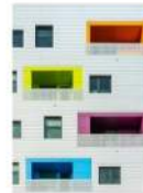
John Pisan Architects - Independence Library and Apartments, Chicago, IL. Photo by James Ferro.
