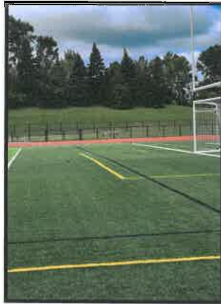
Visible Seams - apparent on all panels
