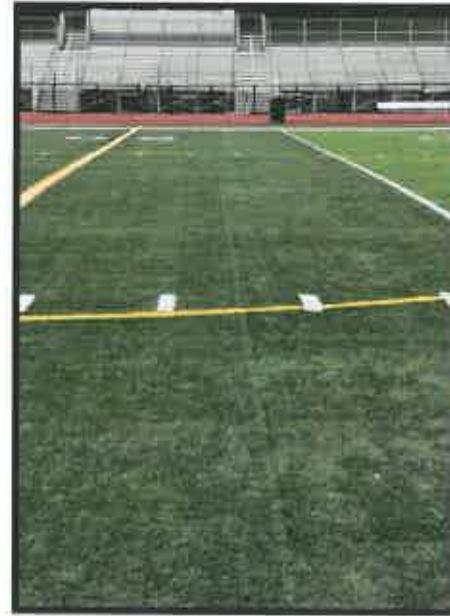
Visible Seams - apparent on all panels
