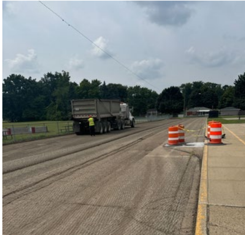
Parking Lot Milling
