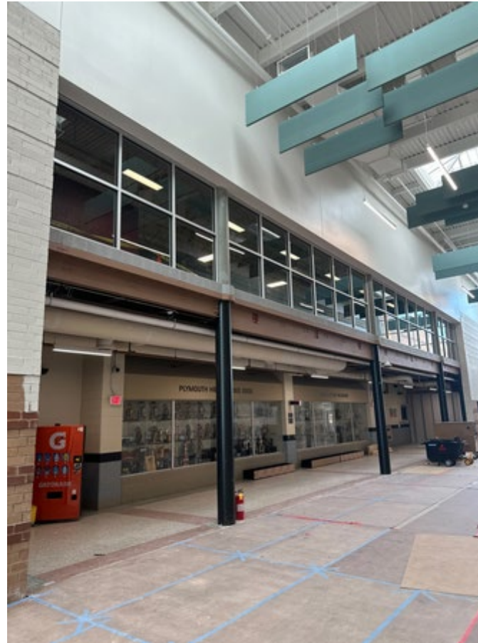
Glass Store Front in Corridor
