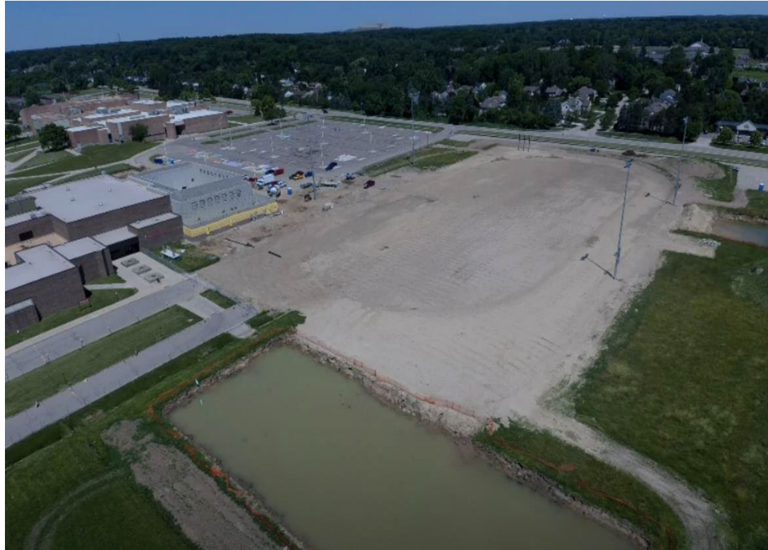
Stadium as of June 2024
