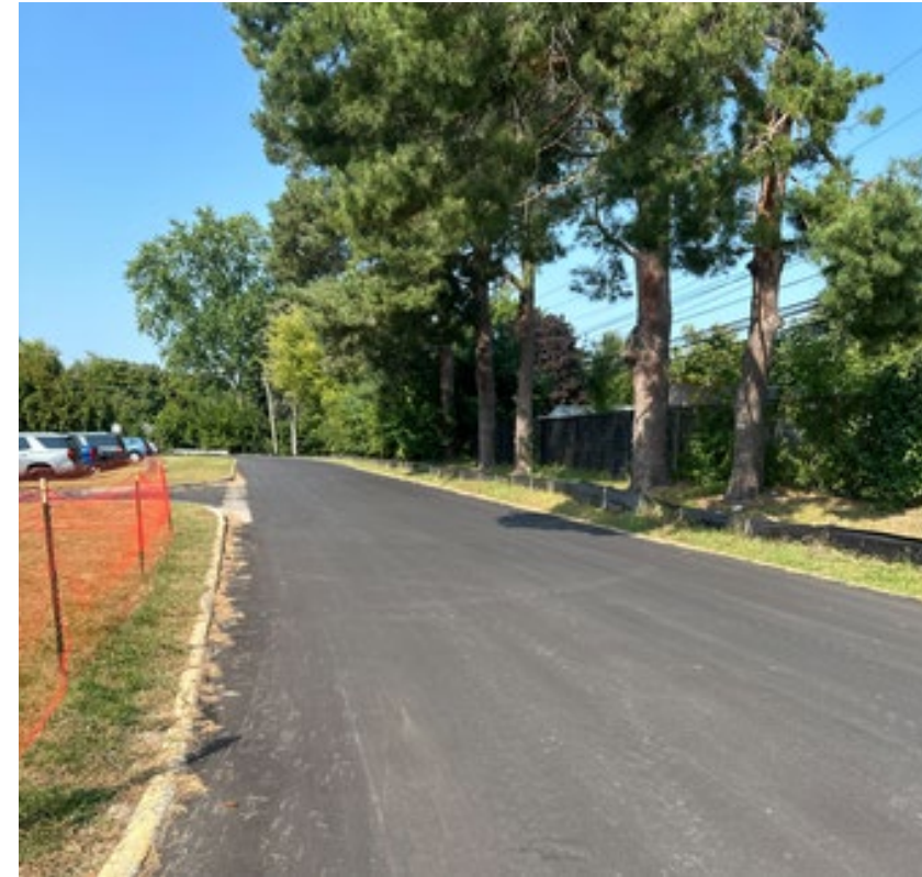
Parking Lot Asphalt
