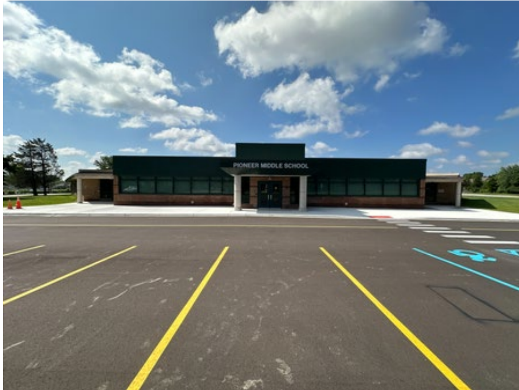
Main Office Addition
