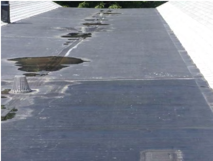
Rubber Membrane Roof
