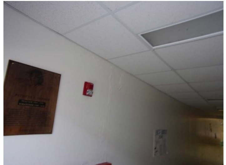
Stress Crack in Hallway
