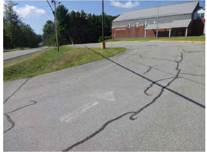
Paving with Sealant
