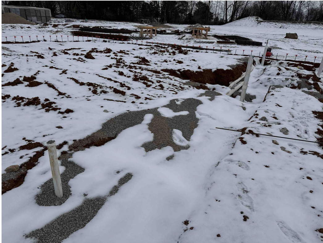
Storm Shelter Under slab Plumping work in Progress
