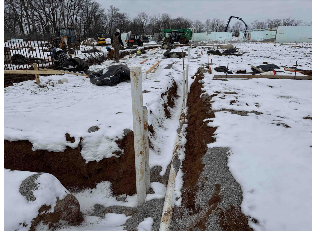
Storm Shelter Under slab Plumping work in Progress
