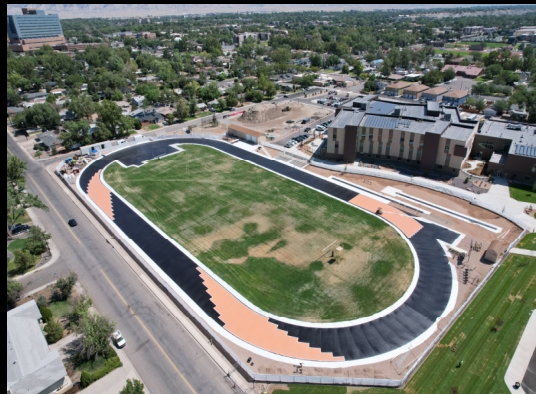
Track Installation Underway
