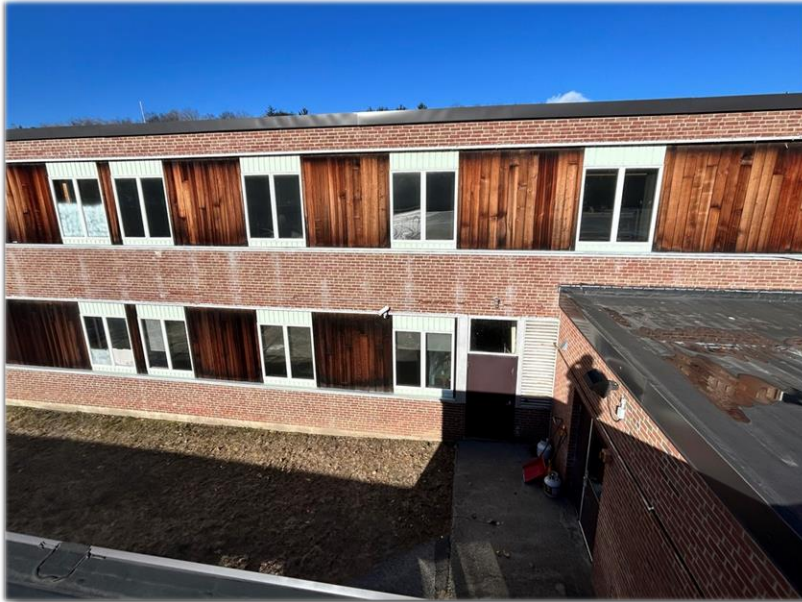
Combustible skin material of RUHS/MS/RTCC - Former original window ban opening
