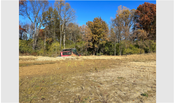
Description Clearing trees along the north property for the permanent drive
