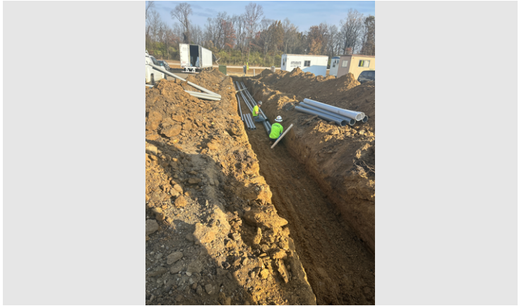
Description Continuing the underground conduits for gas and electric
