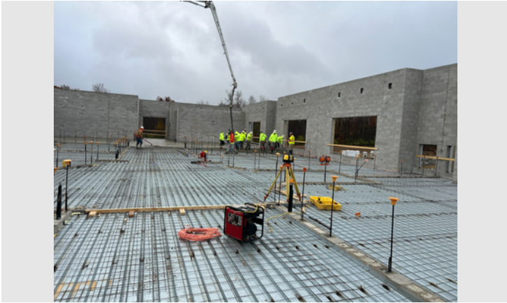
Description Pouring the second floor slab of Zone B - Part 1
