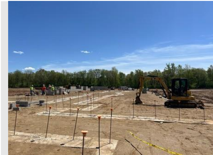
Description: Completed footings and backfill in Area B
