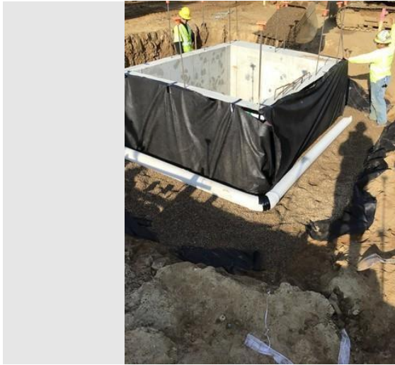
Description: Installing drainage tile around elevator pit
