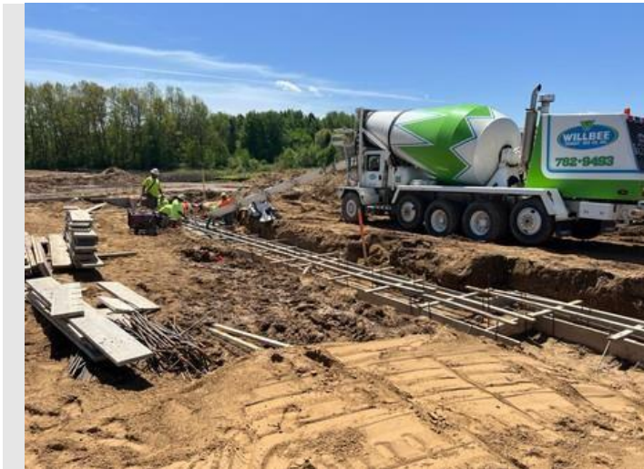
Description: Strip Footings being poured in Area A
