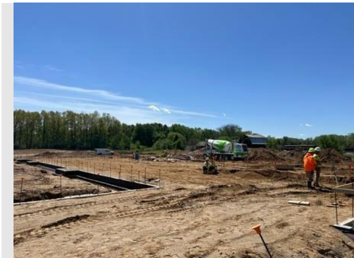
Description: Final footings in Area A
