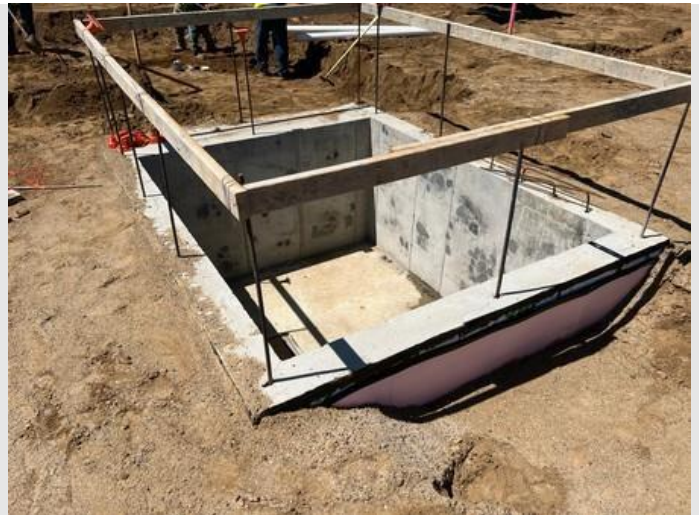
Description: Elevator Pit
