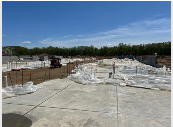
Description: Plastic being removed from Area E floor slabs
