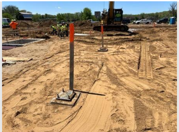
Description: Column anchor bolts in Area C
