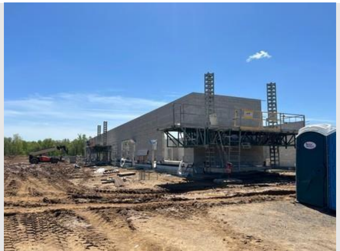
Description: Full height walls in Area F
