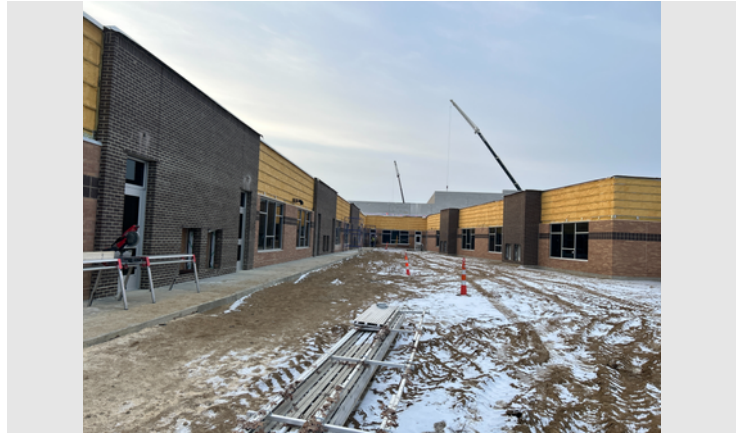
Description Courtyard between Zones E & F.
