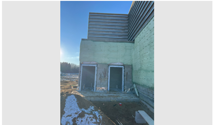
Description Exterior/recess bathrooms on the end of Zone B
