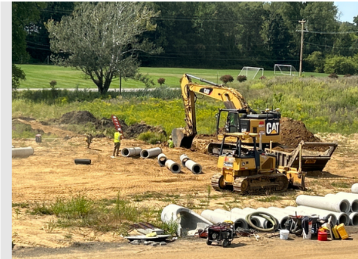
Description Excavation for storm drainage piping.
