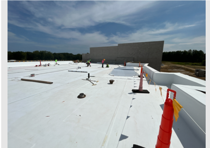
Description Completing the TPO roofing on Zone E
