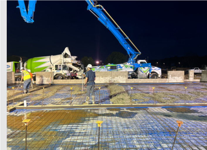
Description Pouring first floor slab in Zone A.
