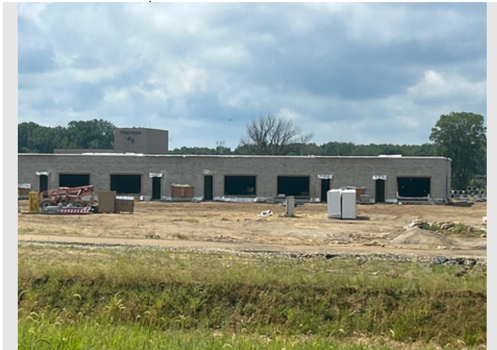
Description East side of Zone F prior to starting brick veneer.
