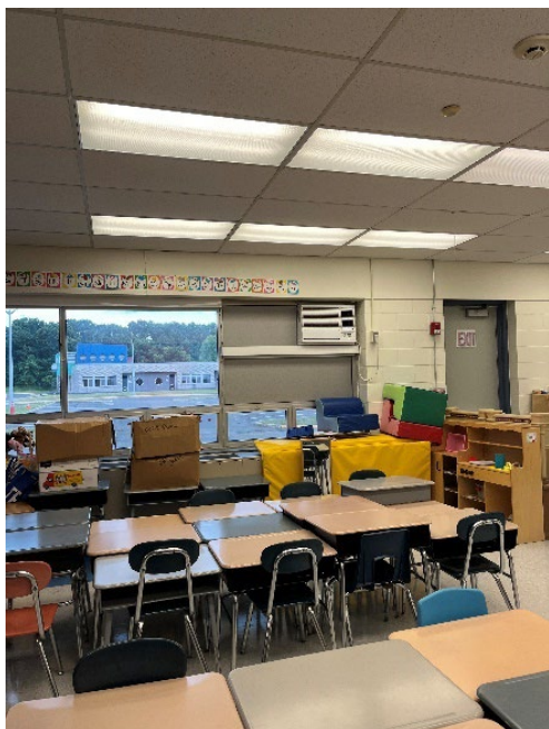
Lighting at Mill Lake School
