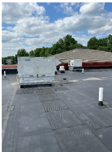
Brookside School – Existing Roof
