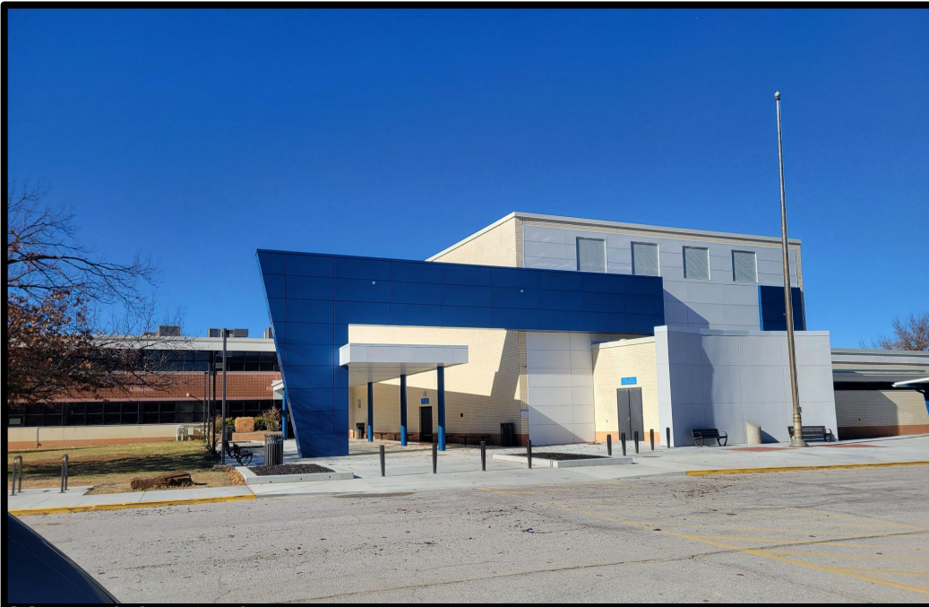
Memorial entry in progress.
