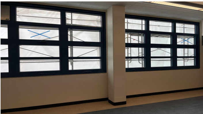
Classroom interior with window replacement
