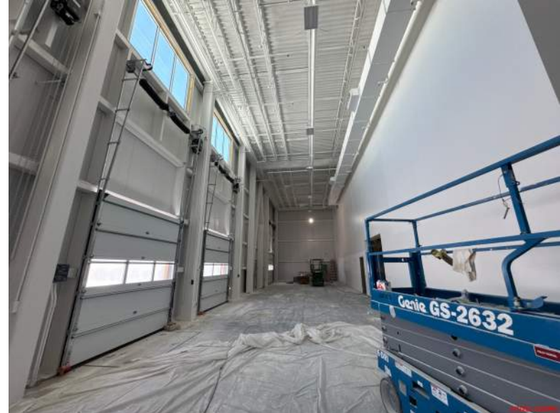
Garage Doors/Ceiling Paint
