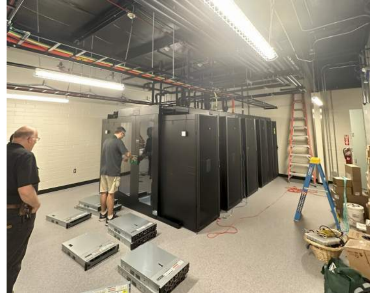
Data Pod Install
