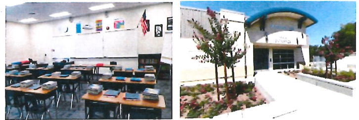
Classrooms after renovation
