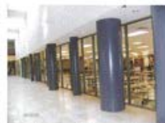
Freshly painted columns building-wide
