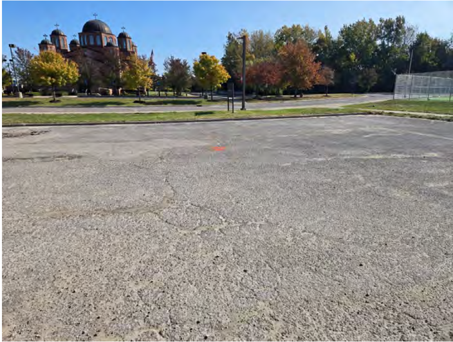
Photograph No. 21: Looking west toward B-68, high severity fatigue cracking
