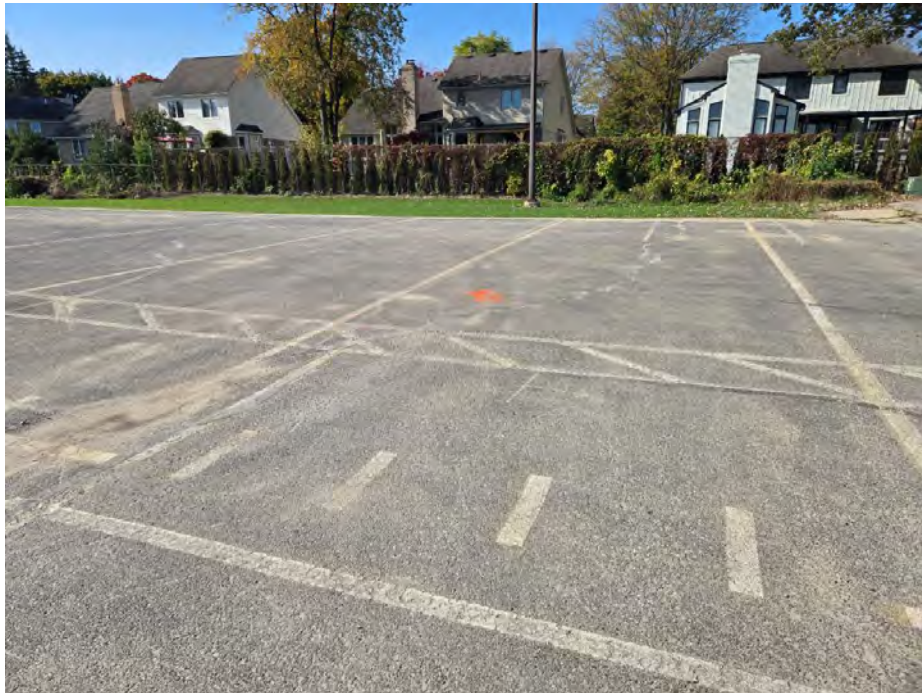
Photograph No. 16: Looking west toward B-64, moderate severity block and fatigue cracking
