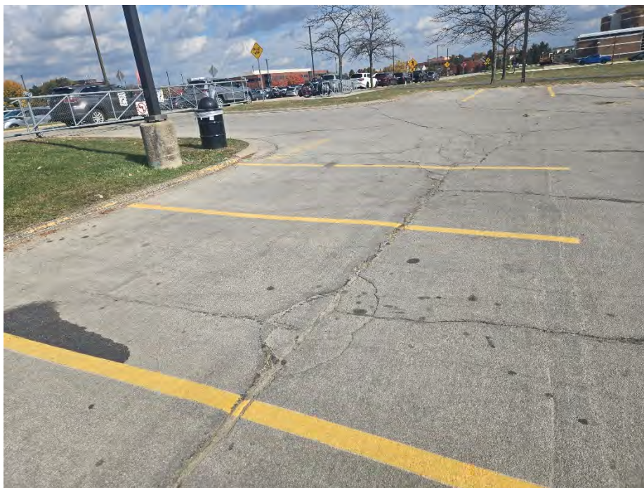
Photograph No. 4: Looking east toward B-5, moderate to high severity fatigue and block cracking
