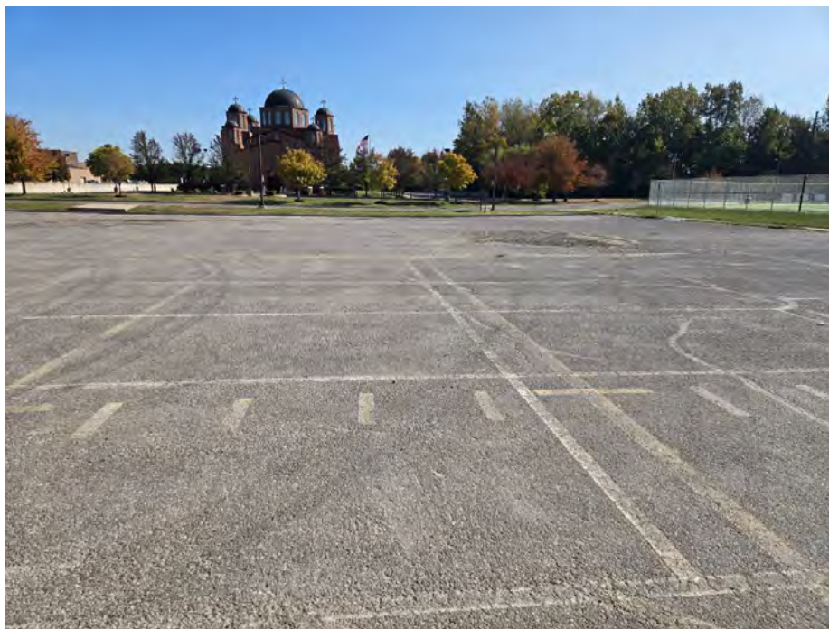
Photograph No. 20: Looking east toward B-68, moderate severity block and fatigue cracking
