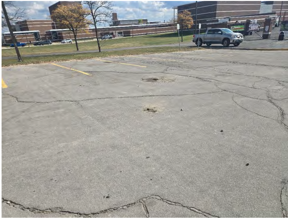
Photograph No. 3: Looking southeast toward B-4, moderate to high severity block and fatigue cracking
