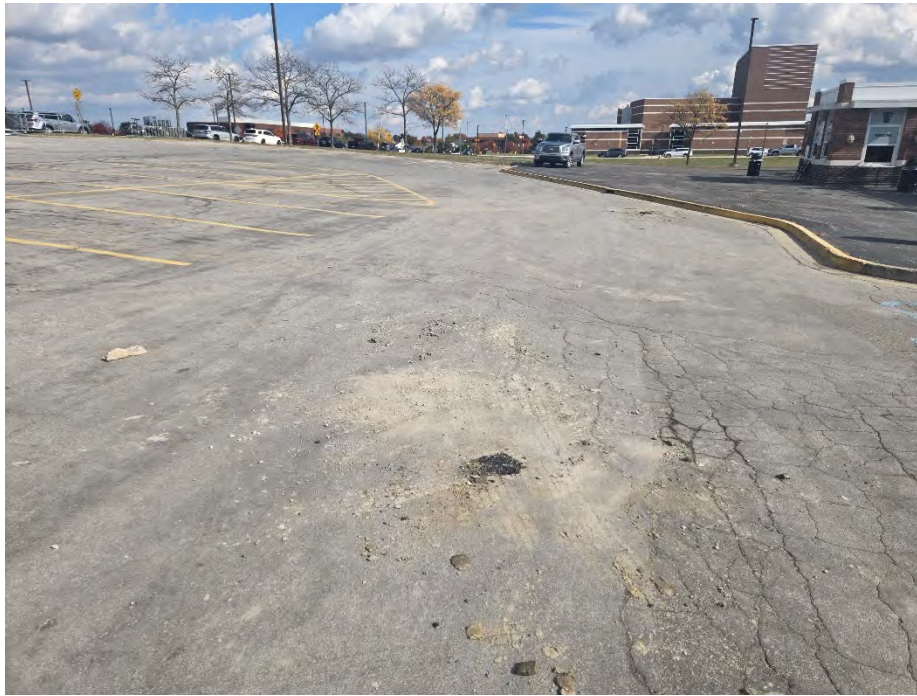
Photograph No. 5: Looking east toward B-1 and beyond, moderate severity fatigue cracking
