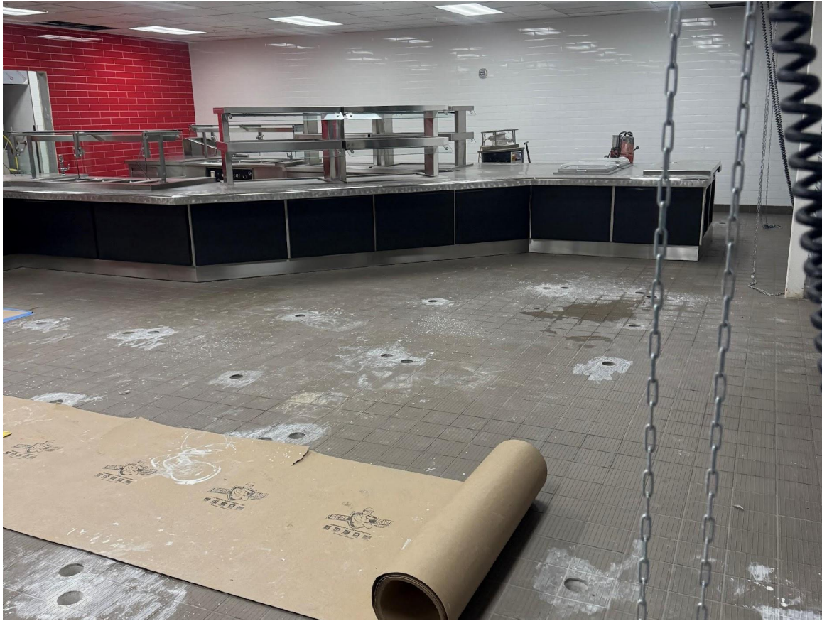
Kitchen Equipment Install
