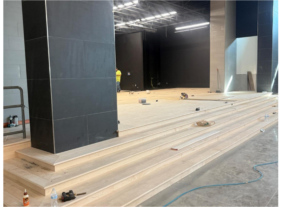
Cafeteria Stage install
