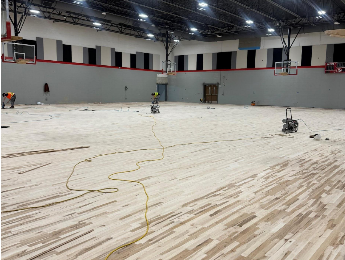
Gym Floor Install
