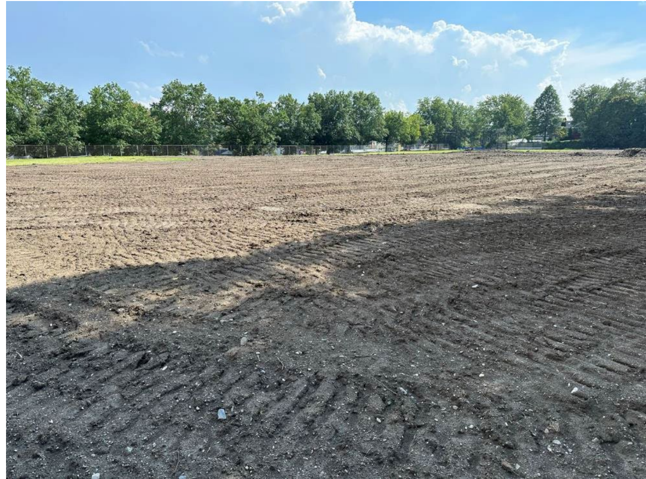
Lawn Restoration Underway
