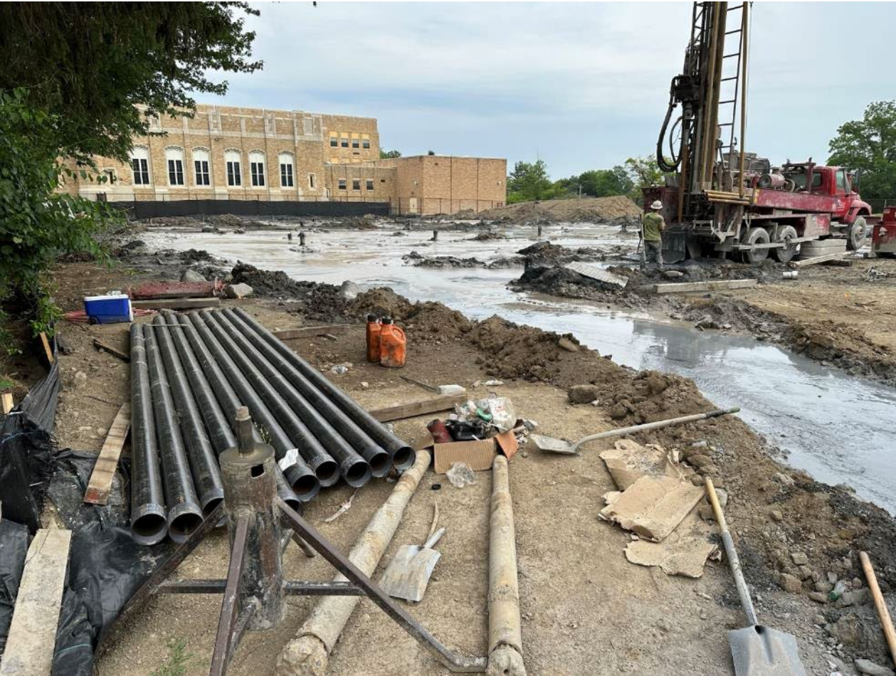
180 Wells Installed Summer 2023
