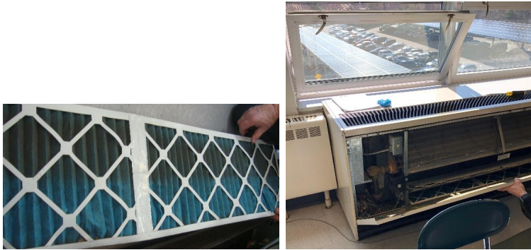
Figure 25 Classroom Unit Ventilators
