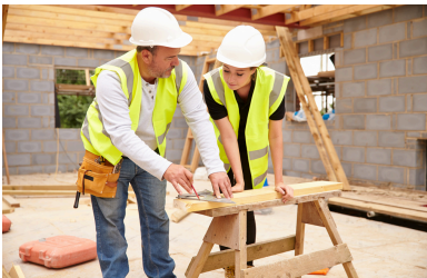
CONSTRUCTION SKILLED TRADES
