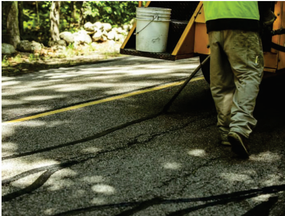
Crack/Mastic Sealing
