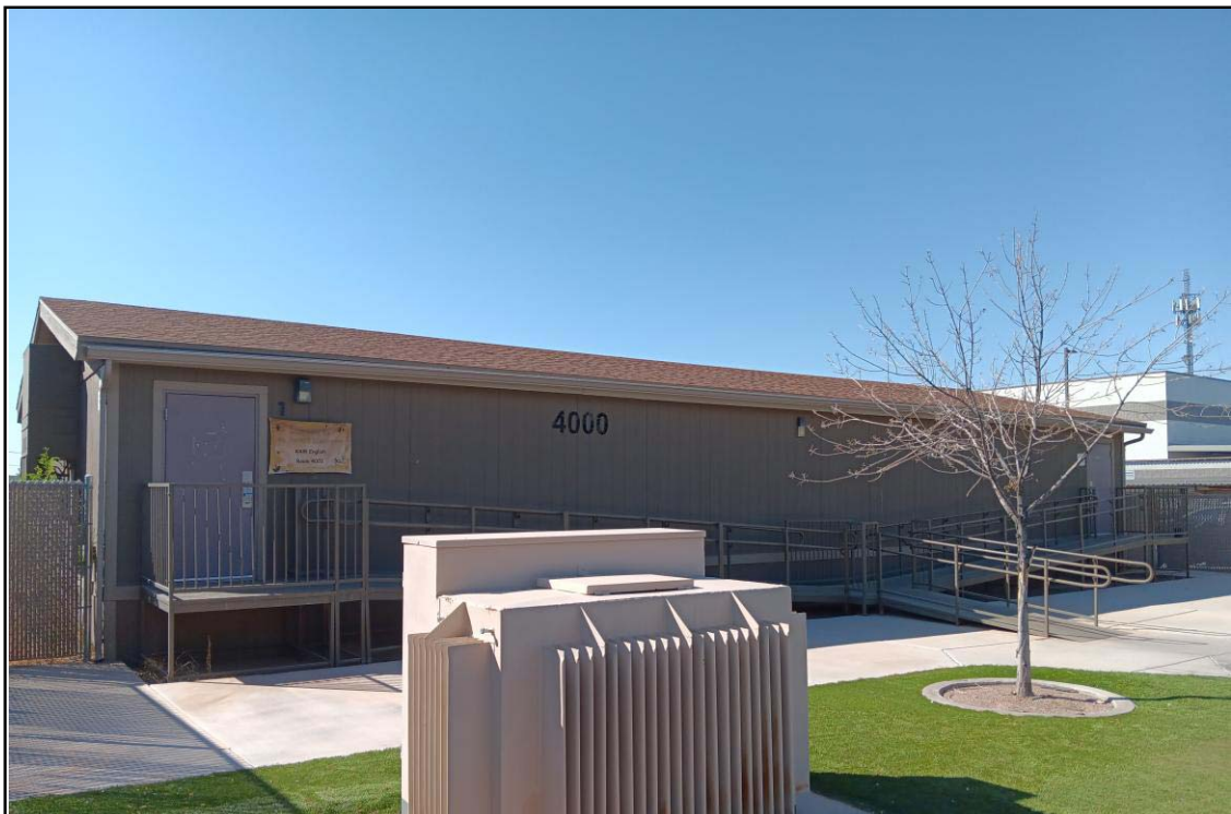
Picture 2 – Building 4000 exterior.
