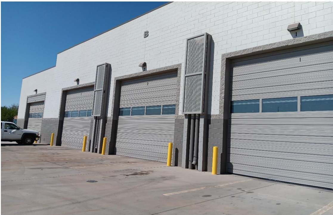
Picture 2 – Garage warehouse entrance.
