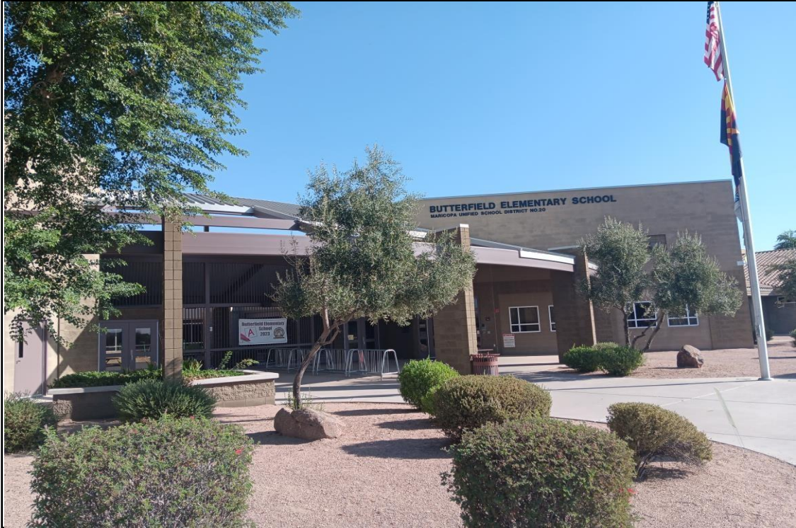
Picture 1 _ The front entrance to Butterfield Elementary School.
